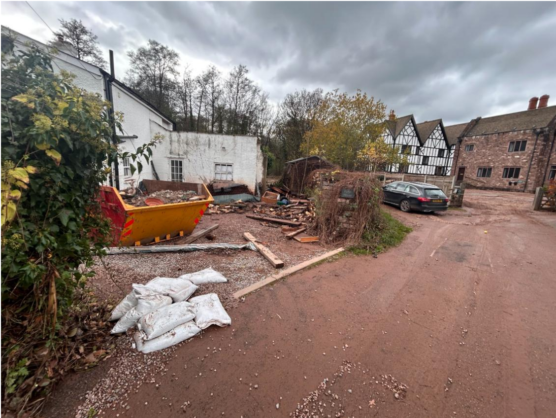
Figure 7-2 Aftermath of Flooding within Forge Road Study Area
