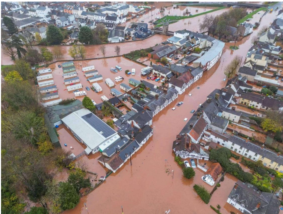
Figure 8-5 Drone Image of Flooding Across West of Monnow Study Area
