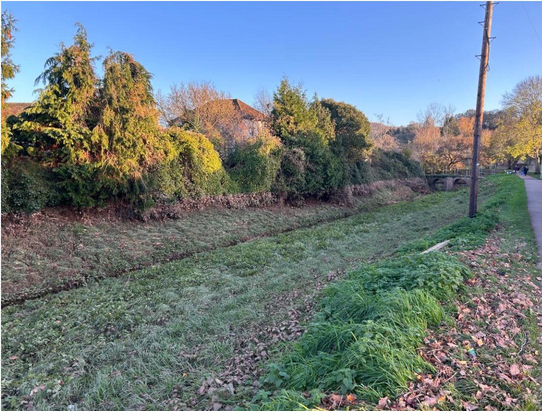
Figure 8-9 Flood Level within Old Town Ditch
