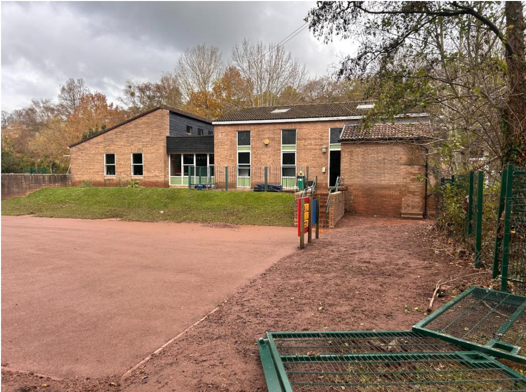
Figure 9-3 Osbaston Primary - Water Level Mark
