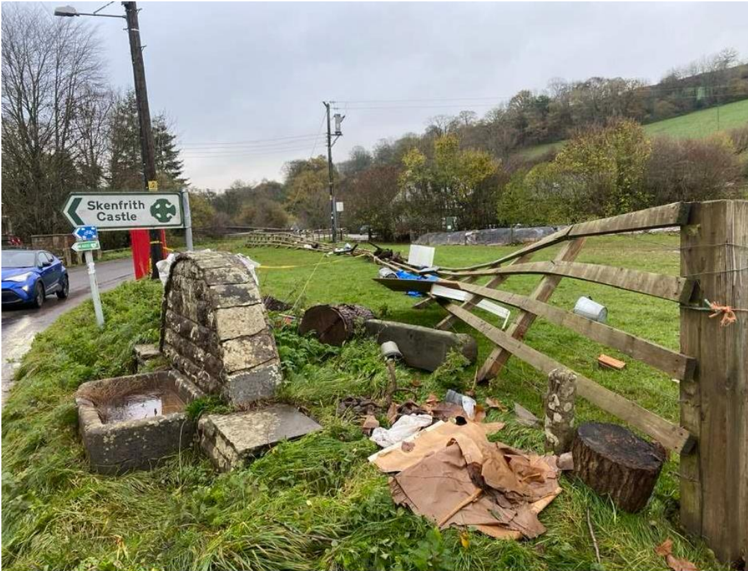
Figure 5-2 Flood Flows Resulted in Damage to Fencing
