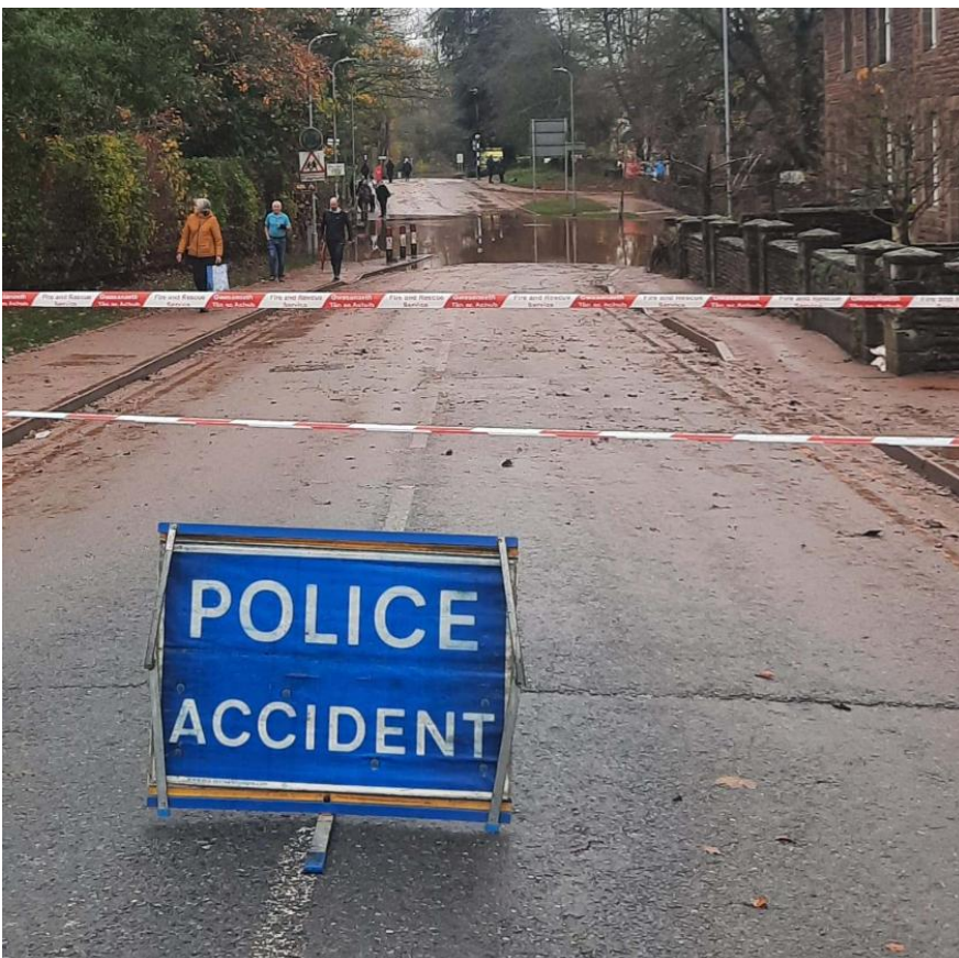
Figure 8-16 Aftermath of Flooding along Watery Lane
