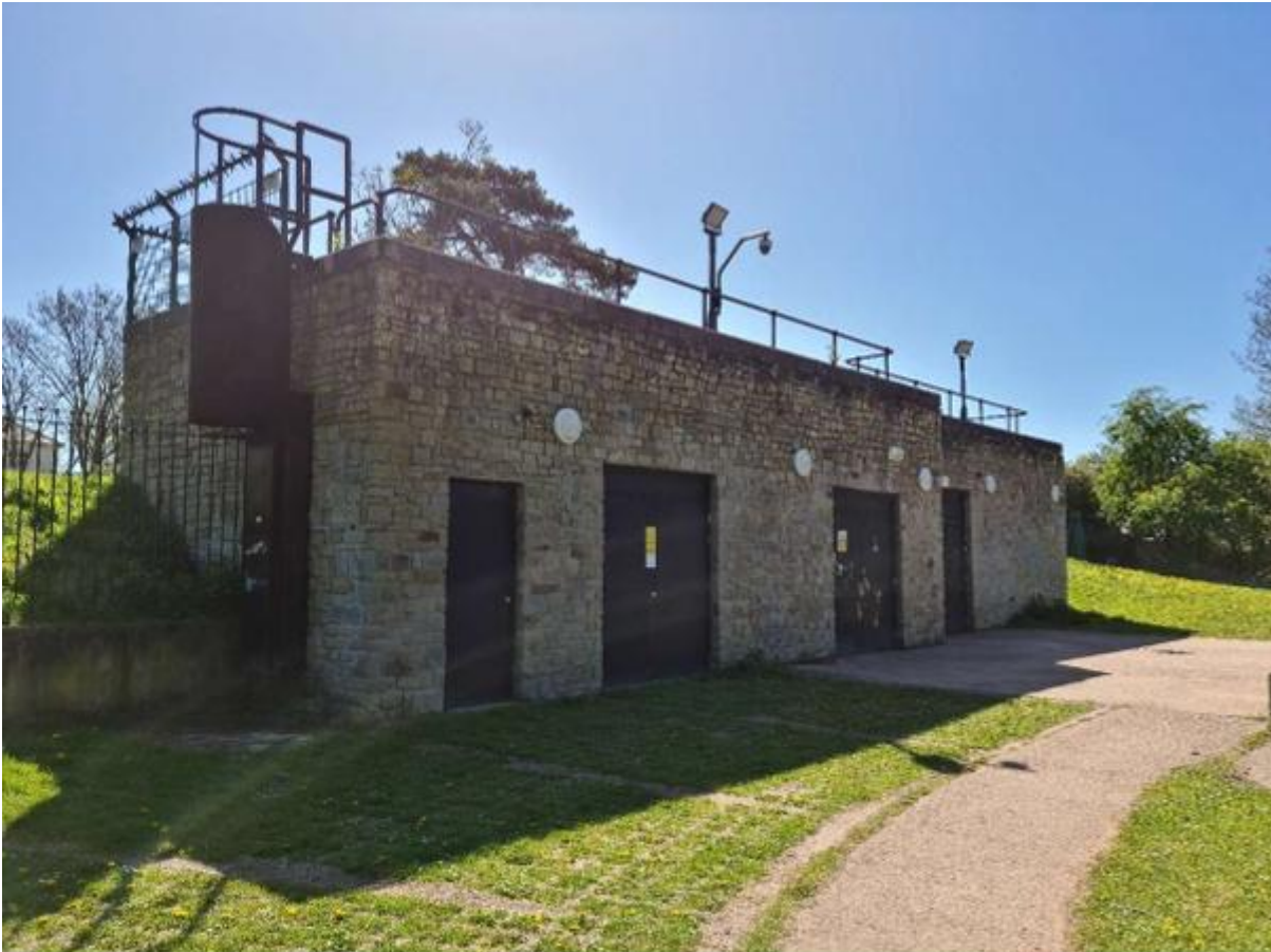
Figure 3-2 Wonastow Road Flood Alleviation Scheme pumping station
