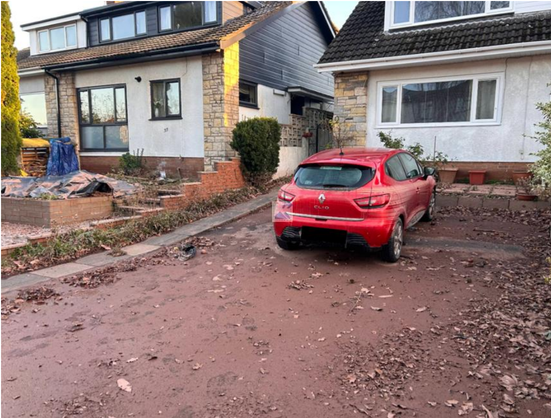
Figure 8-11 Evidence of Water Level, Wonastow Road
