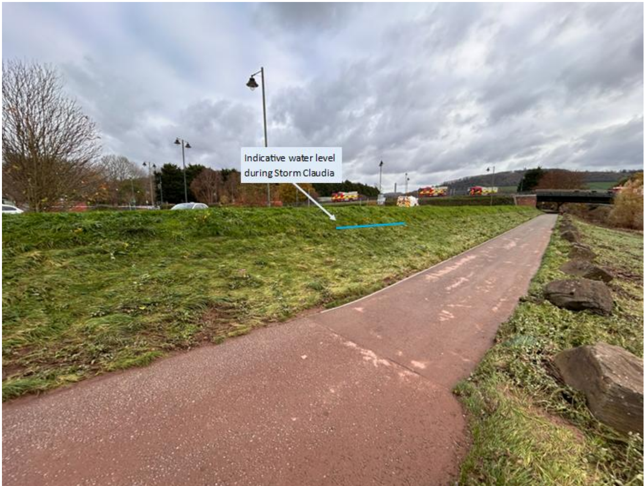
Figure 8-8 Evidence of Water Level Downstream of Monnow Bridge
