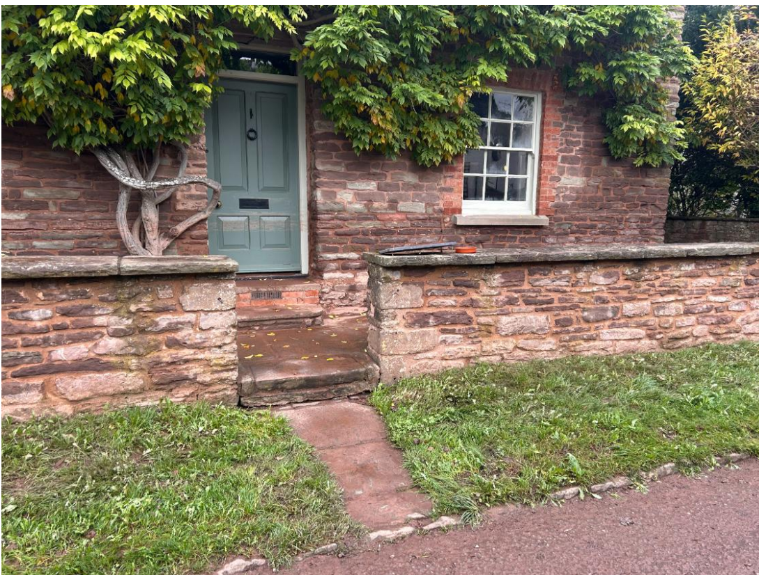
Figure 5-5 Evidence of Water Level on Property
