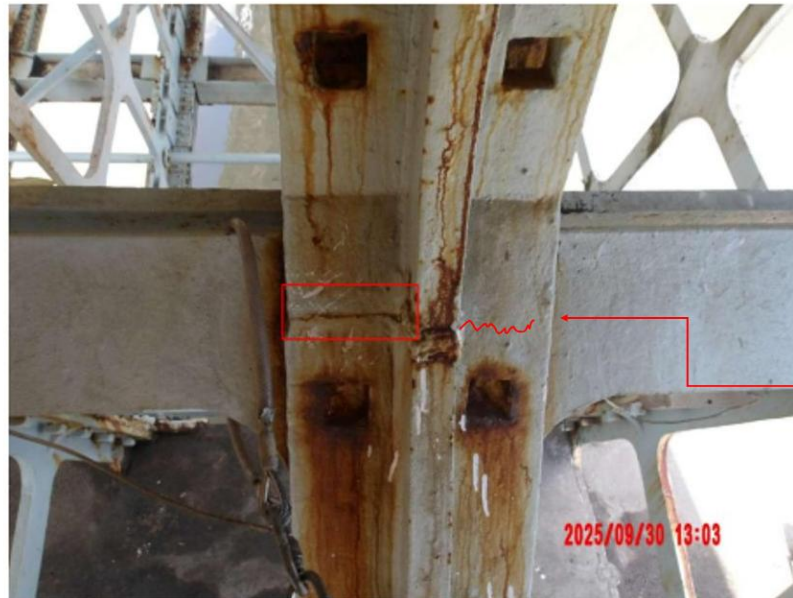
Existing crack propagating
