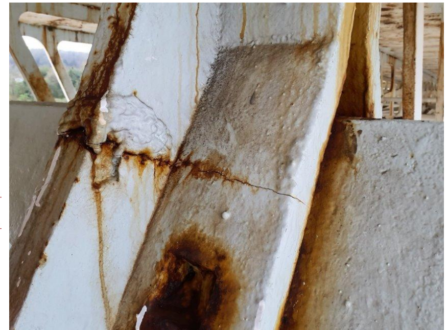
Existing crack propagating
