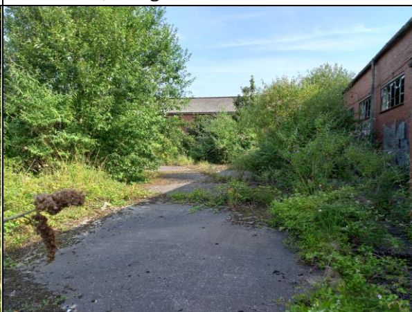
Photo EDP 8: Hardstanding surrounding the derelict buildings with encroaching scattered scrub, facing north.
