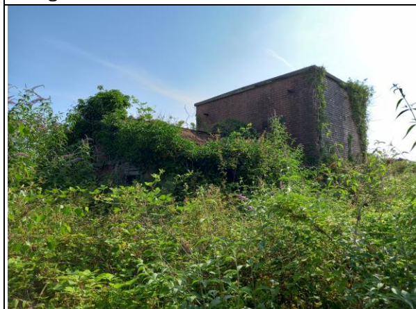
Photo EDP 9: Building B2 with confirmed lesser horseshoe maternity roost, surrounded by dense scrub, facing north-west.
