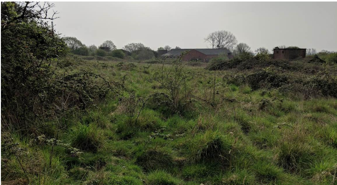
Image EDP 2.1: The site comprises several derelict buildings within the centre of the site.
