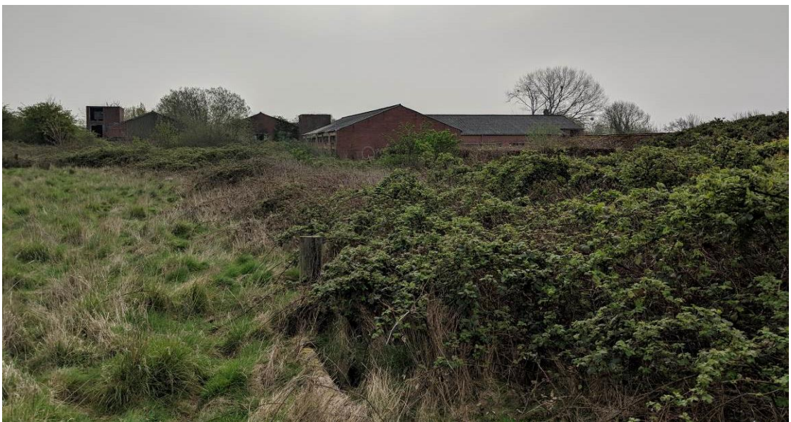
Image EDP 2.2: The site comprises several derelict buildings within the centre of the site.
