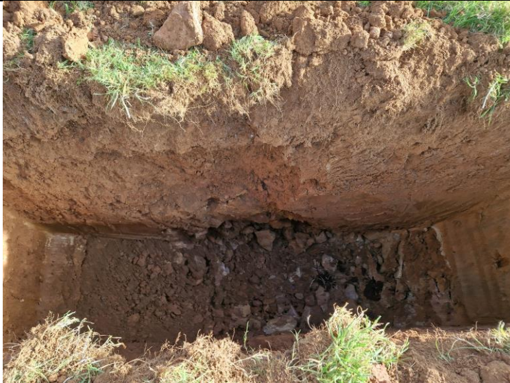
PLATE 09 – Trial Pit Excavation – TP05.
