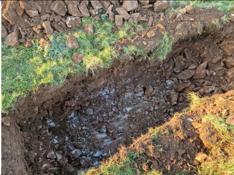
PLATE 05 – Trial Pit Excavation – TP03.
