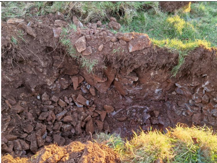
PLATE 07 – Trial Pit Excavation – TP04.
