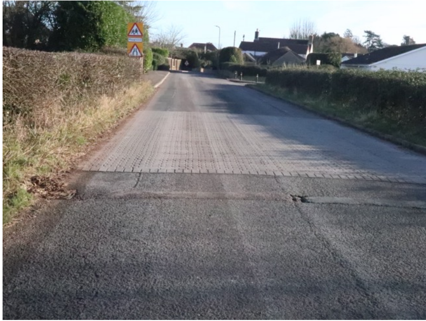
Figure 5 Textured Surfacing on Earlswood Road
