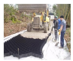
and traditional aggregate and geo grid-reinforced structures demonstrate a 50% reduction in construction thickness of the granular material.
