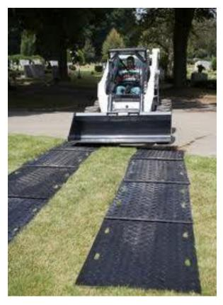
The use of ground protecting boards such as these seen in the adjacent picture should be used. Geo textile and felt may be required beneath these routes to minimize puddling of the soil surface. Should puddling occur, a capped layer may well be formed which will reduce the lateral diffusion of soil gasses and cause significant problems for retained trees.
