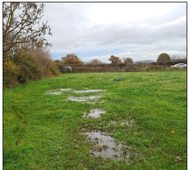
Figure 6 - Area of Standing Water Following Rainfall.
