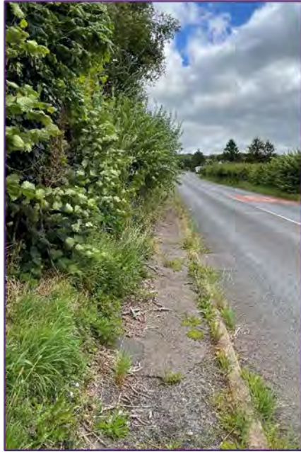
Monmouth Road footway to east of the Site
