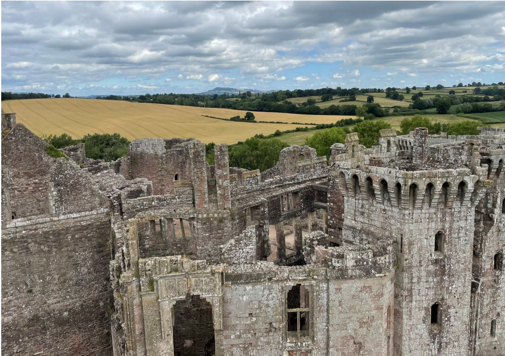
Plate 5: North-west view from the Great Tower.
