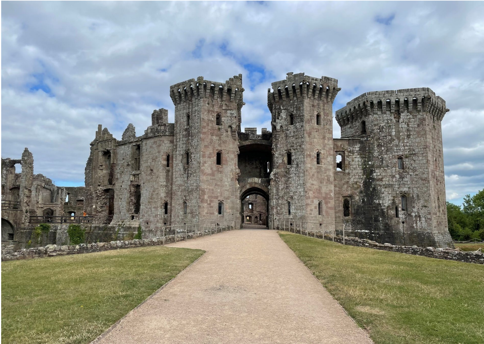
Plate 2: General view of the gatehouse range.
