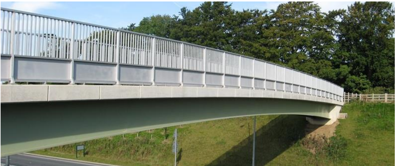
Figure 5-5 – Case Study – Steel Girders with Concrete Slab
