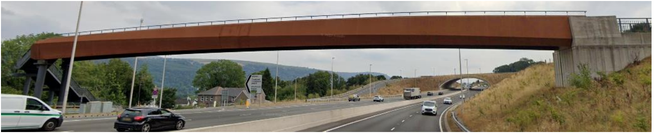
Figure 5-4 - Case Study – A465 Gilwern Structure 15
