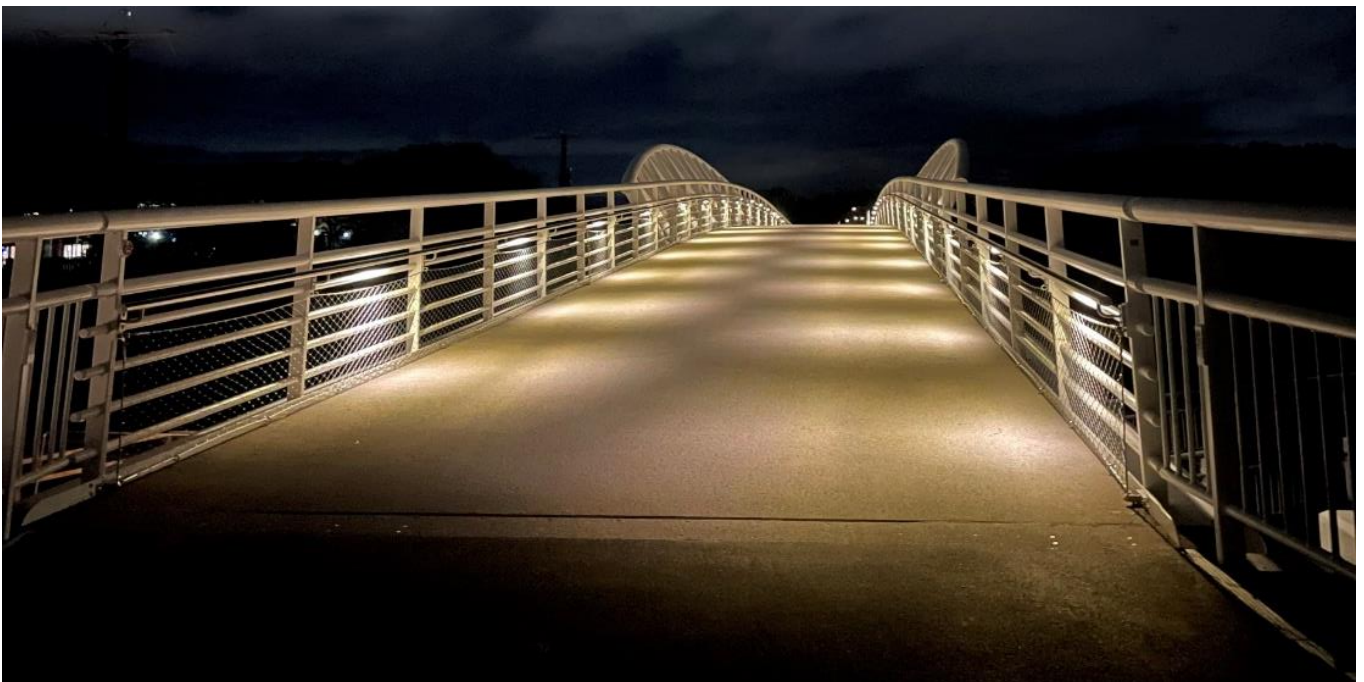
Figure 5-1 – Case Study - Recently Completed Structure (Carmarthenshire County Council)
