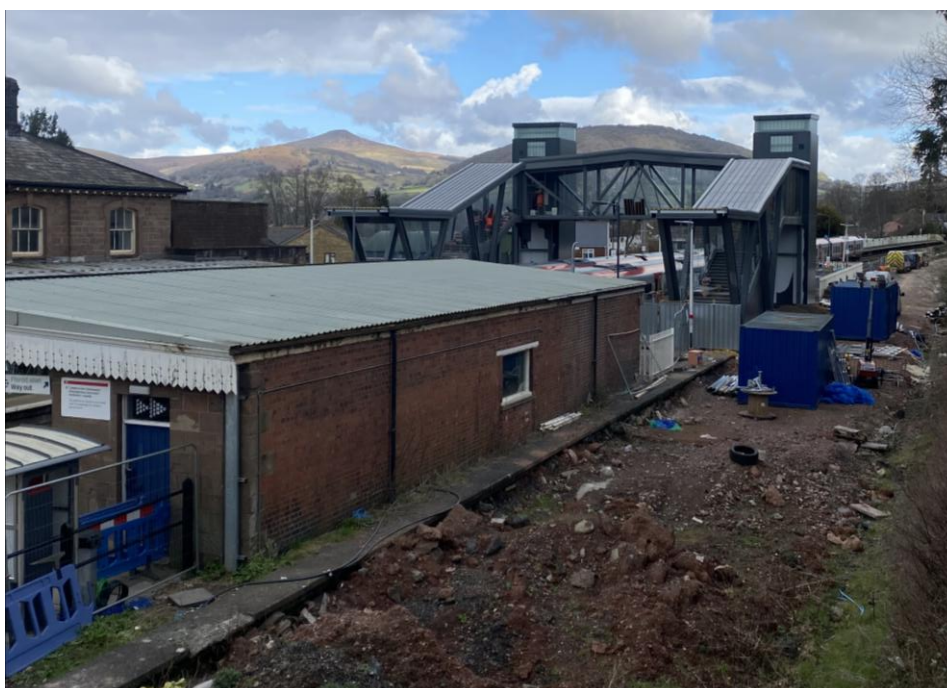
Figure 3.3 'Access for All' bridge at Abergavenny Station
