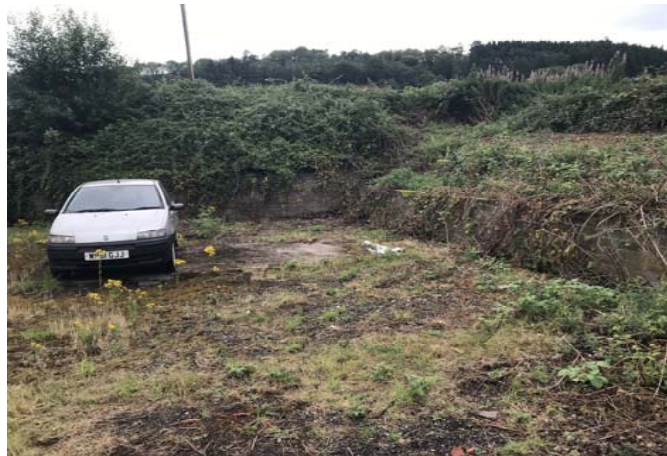
8. Looking east towards retaining wall at Roc House Farm
