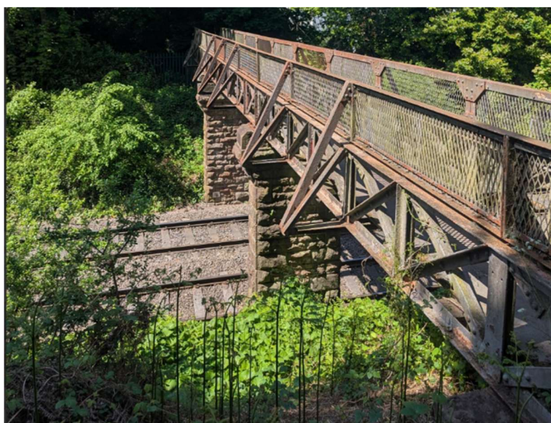
Figure 11 – View of Caederwen Footbridge from A465 End
