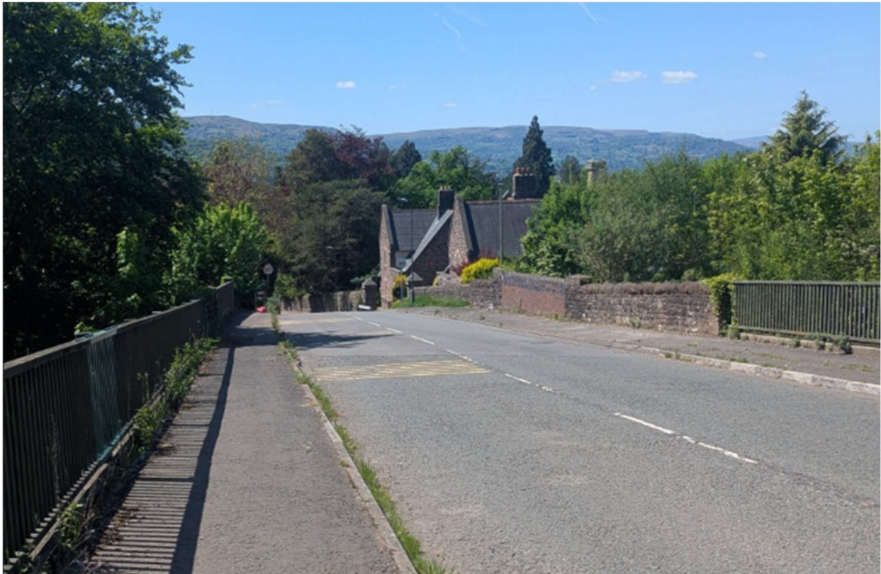
Figure 13 – B4233 Highway Structure from End of Garth Farm Access Road
