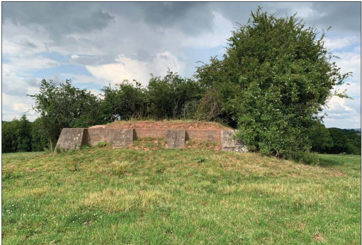
Plate 5 - Concrete structure within northern field, looking north
