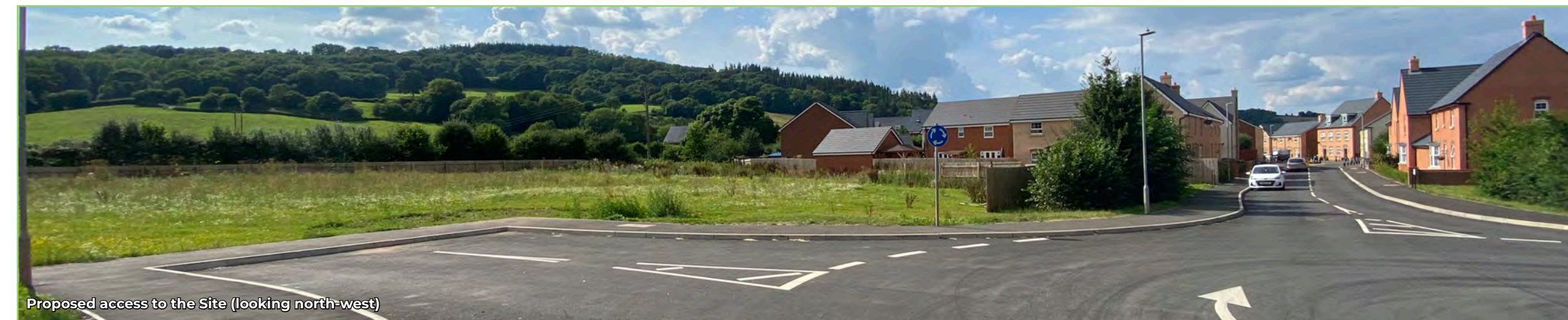
Proposed access to the Site (looking north-west)
