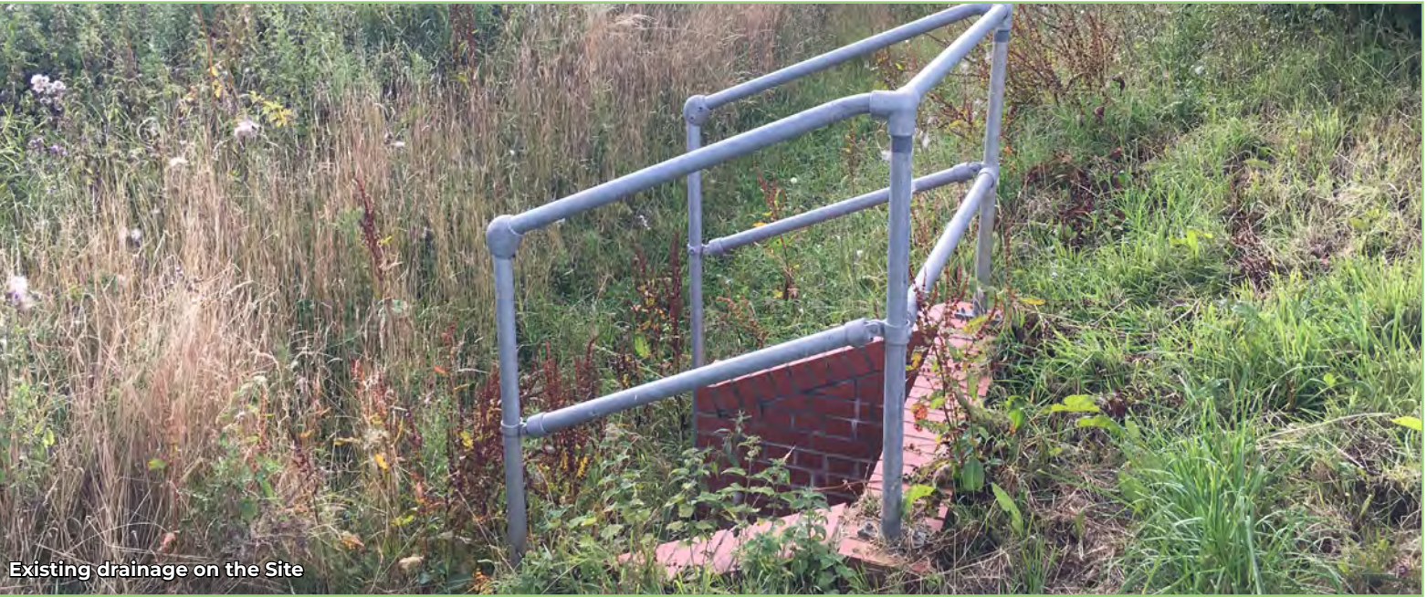
Existing drainage on the Site
