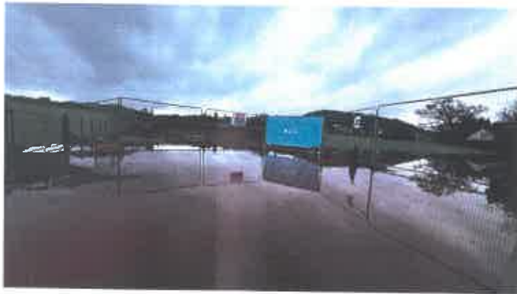
Resident Photo taken Feb 2024 about 24 hours after heavy rain Note the red clay colour of the runoff water
