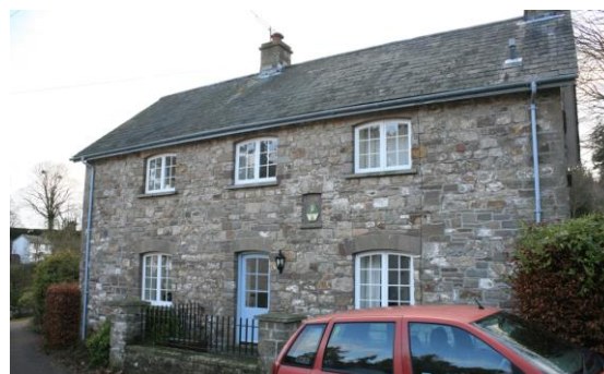
Fig.57 Rhyd-y-Meirch. A larger cottage situated parallel and behind the Post Office Cottages. The skilful use of stone voussoirs forming elliptical arches over the window heads is apparent.
