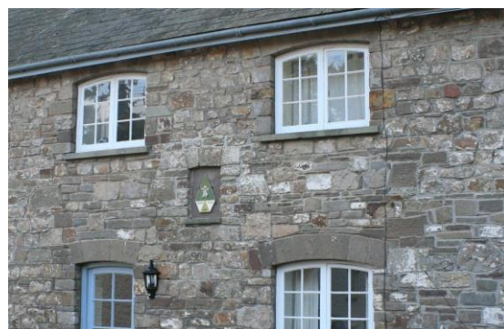
Fig.69 Rubblestone walling is the characteristic material of 19 th century and earlier houses within the Conservation Area
