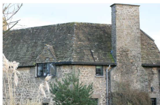
Fig.70 Sandstone is a feature of the vernacular revival houses either squared or as seen here as rubblestone
