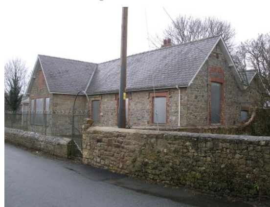
Fig.52 The former Village School: this robustly detailed late Victorian building is now used as a nursery
