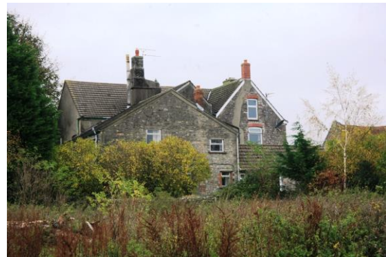
Fig.20 The prominent roof slopes of Great House farmhouse with modern concrete interlocking tiles
