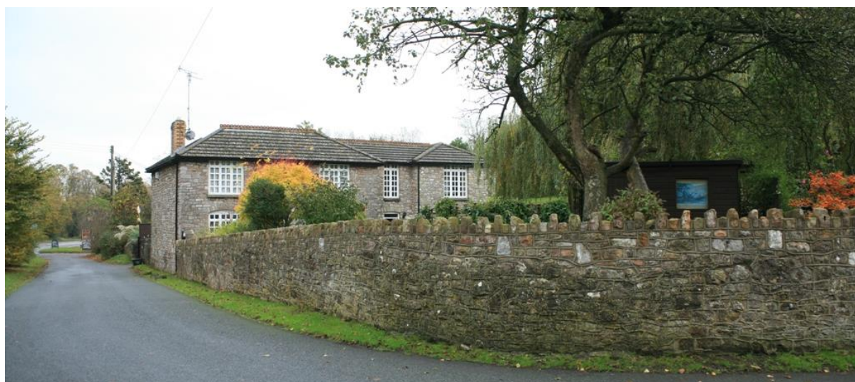
Fig.43 Green Lane with its large multi-pane casement windows, an unusual feature in the Conservation Area
