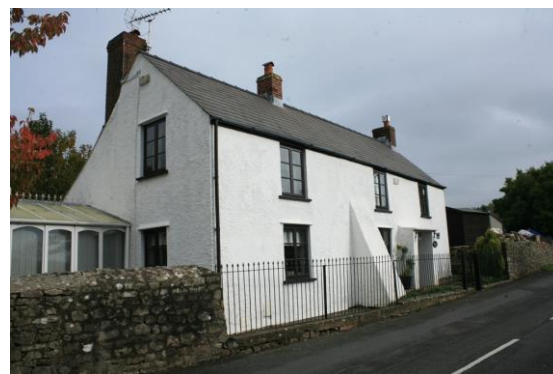
Fig.59 White painted render and natural slate roof, seen throughout the Conservation Area
