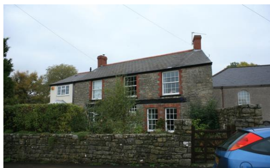
Fig.58 Stone laid to courses with red brick dressings and brick chimneys (Byeways, Pound Lane)
