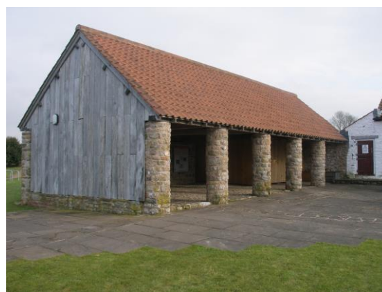
Fig.55 The recently, sensitively converted buildings providing a visitor facility and information point
