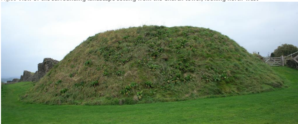
Fig.61 View of Roman town wall and Norman motte from the south
