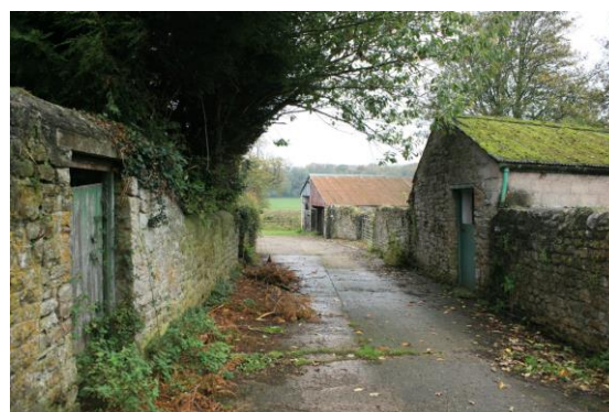
Fig.18 Series of stock yards with low stone buildings and walls enclosing them (Great House Farm)
