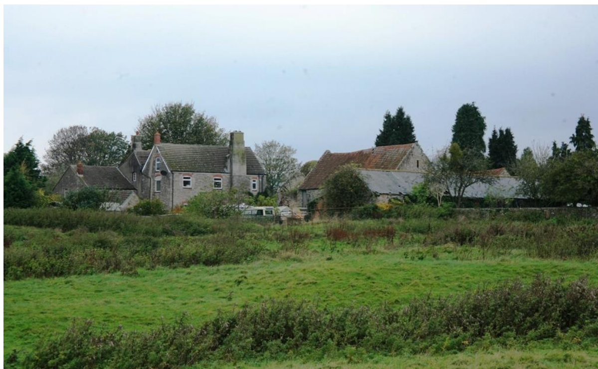
Fig.17 Great House farmhouse and its farm buildings form a group of some considerable local architectural and historic interest
