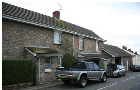
Fig.30 uPVC windows, modern roof coverings and removal of chimneys have eroded the character of the buildings in this part of the Conservation Area – compare this image with the historic photograph at Fig.57 in section 7.5
