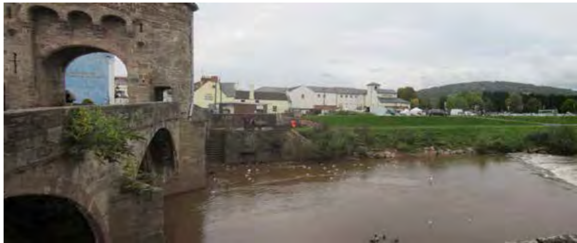
② Views to Monnow Bridge, River Monnow and surrounding hills from St Thomas's Square approach
