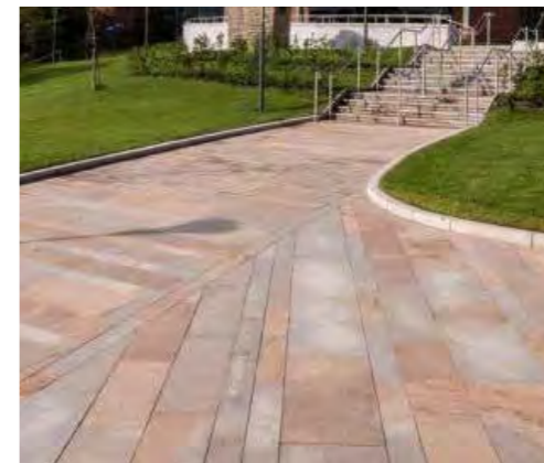
Red granite paving - Steps
