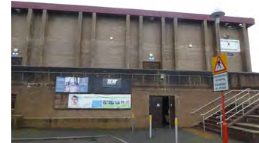
Chepstow Leisure Centre Exterior
