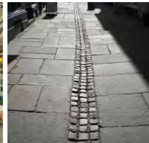
The small streets in the historic core are characterised by a high quality floorscape of Pennant stone flags and central gully of small stone setts.
