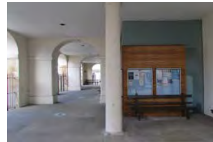
Current screens to entrance foyer do not allow view to the inside from some angles
