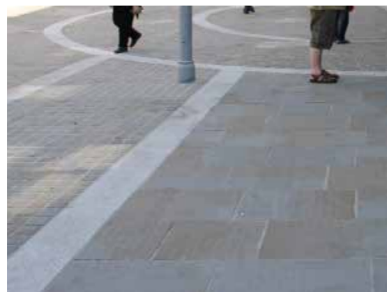
Pennant stone paving - sawn and flame textured bands
