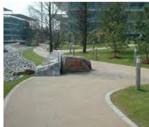
Resin bonded gravel riverside paths
