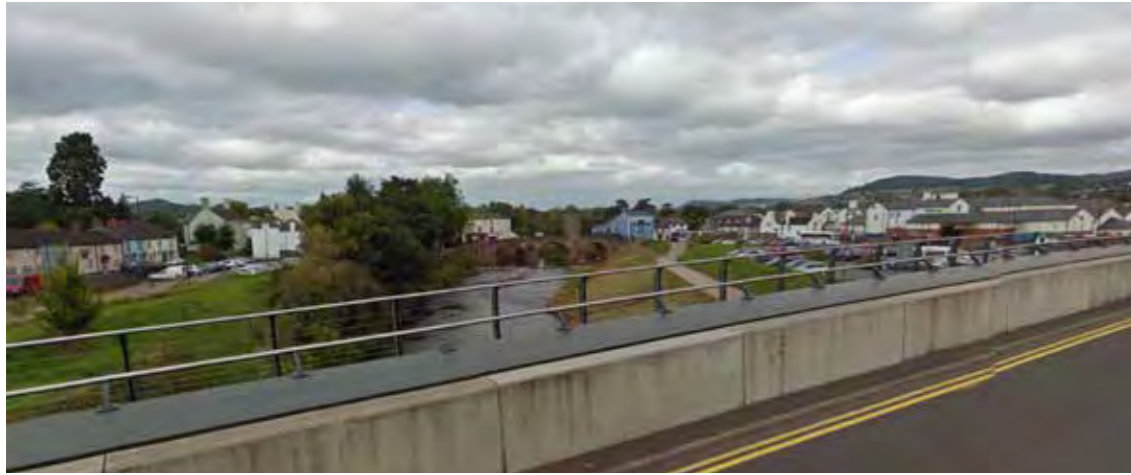
① View from new bridge obstructed by bridge balustrade
