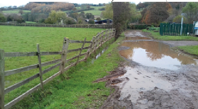
Rear track to Orchard Close. Small right-hand ditch conveys water to piped drainage system.
