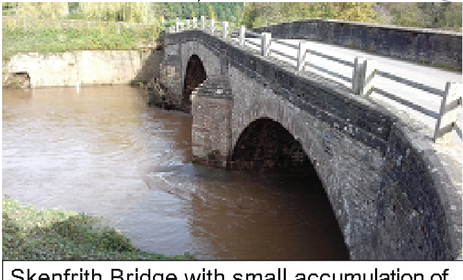
Skenfrith Bridge with small accumulation of debris on cut water after flood event
