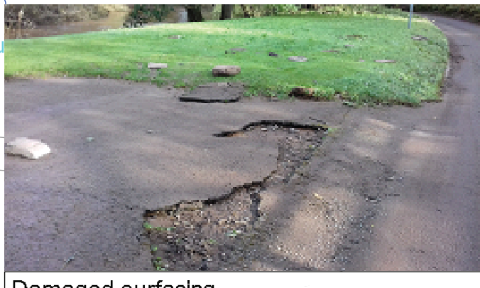
Damaged surfacing
