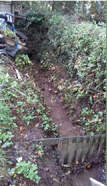
Open channel from surrounding fields to culvert beneath the C12.13 carriageway. Inlet protected by private homemade screen.
