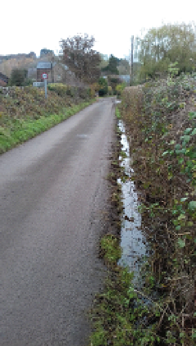
Roadside ditch looking downstream towards connection with piped drainage system
