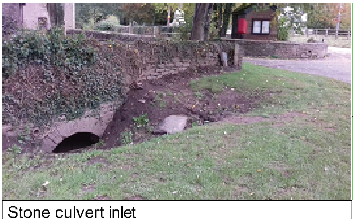
Stone culvert inlet
