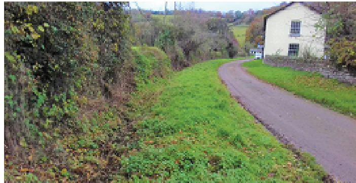
Roadside ditch along left hand verge looking upstream towards Dry Bridge (Malthouse on left).
