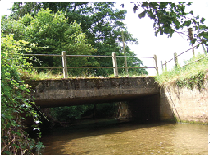
Downstream elevation at Dry Bridge which carries the C12.13 over the Norton Brook
