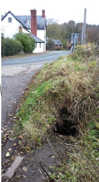
Culvert inlet / open chamber
