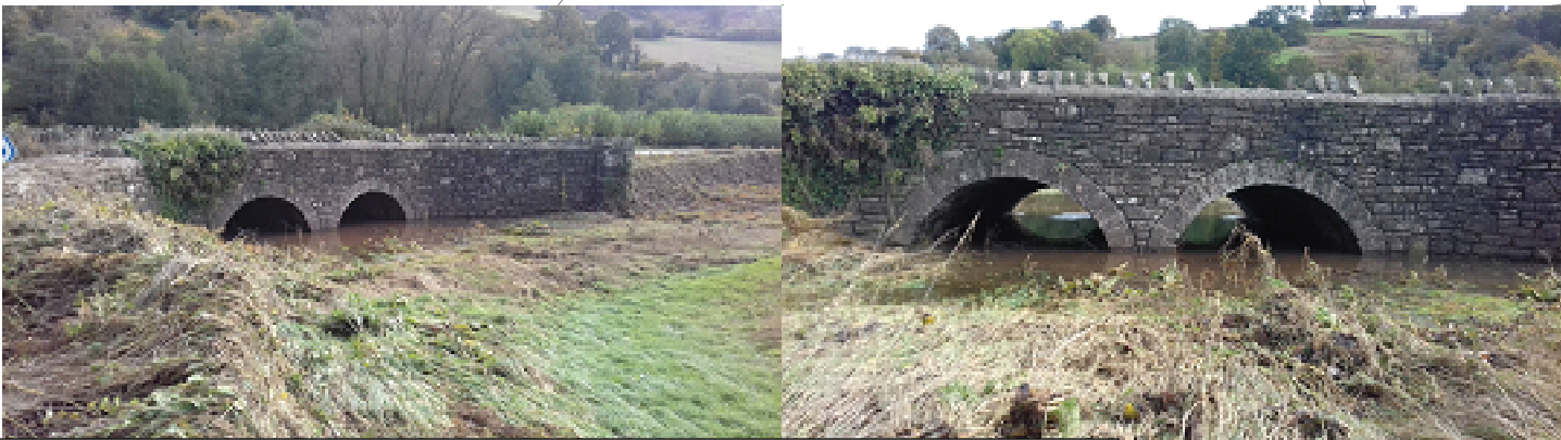
Downstream elevation of masonry flood relief arches.
