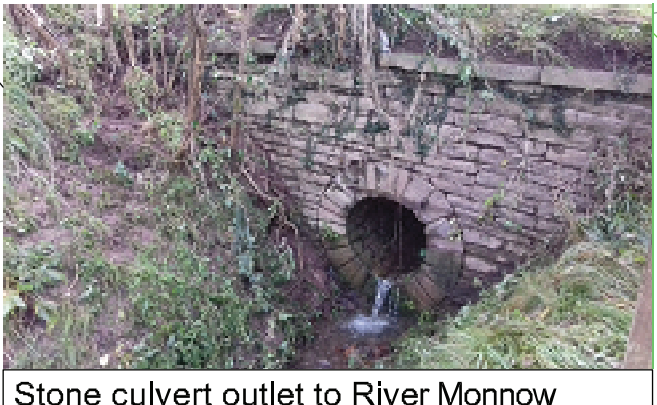
Stone culvert outlet to River Monnow
