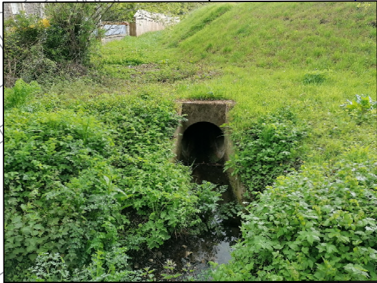
Culvert Inlet at Usk Island
