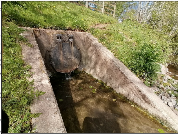
Culvert outfall headwall & flap valve
