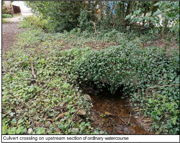
Culvert crossing on upstream section of ordinary watercourse
