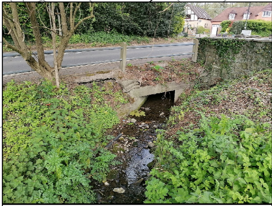
A472 Culvert Outlet
