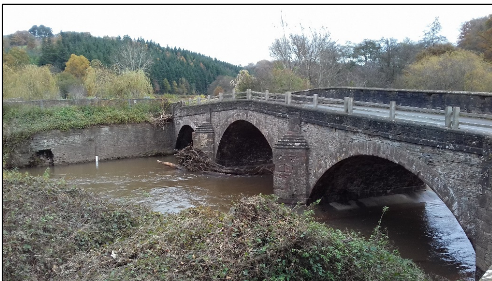
Photo 2: Skenfrith Bridge with a small accumulation of woody debris on the far cutwater post event
