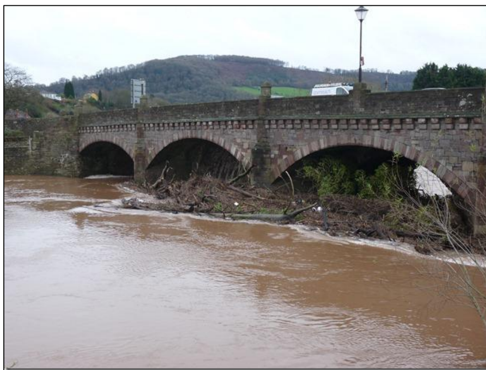
Photo 13: Debris build up on the upstream side of Wye Bridge as a result of the flood event
