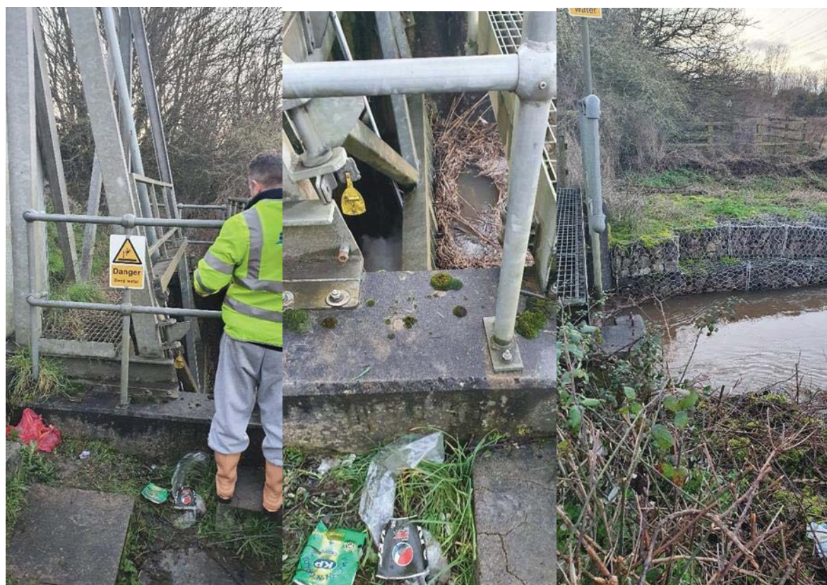
Photos 15, 16 and 17: Shows Highways England staff at the Trash Screen in March 2020 also showing some of the Debris
