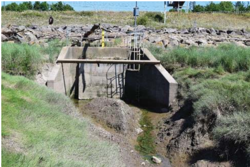
Photo 20: The Sea Door where the Neddern Brook Outfalls and Shows Silt Deposit in Front of Door taken June 2020
