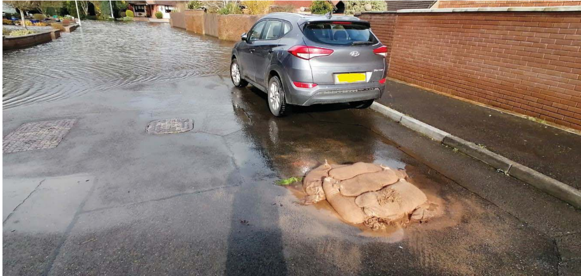
Photo 2: Showing the Surcharging Surface Water Manhole at Castle Lea, taken on 1 st March 2020
