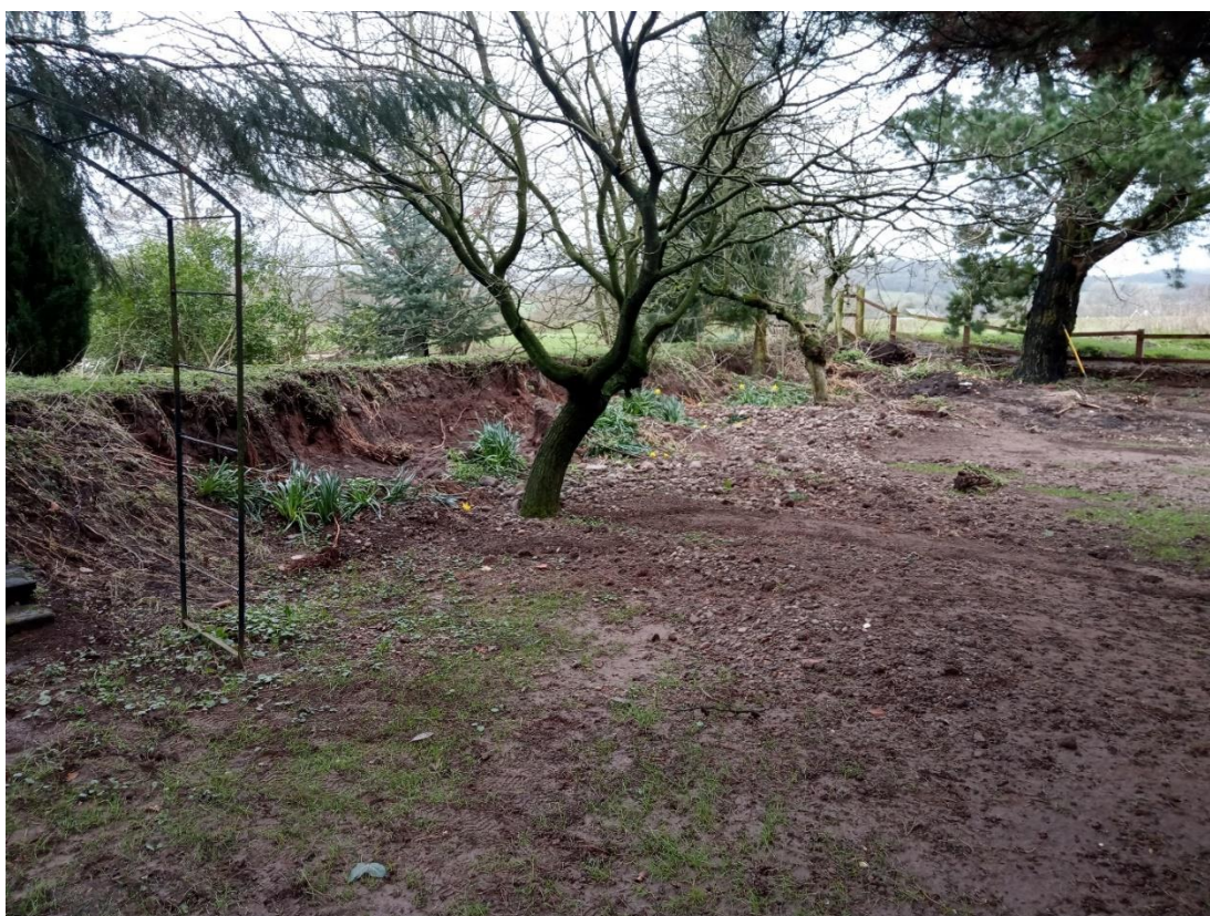
Figure 12 - Damage to rear of Flood Defence Embankment, Llangronwn
