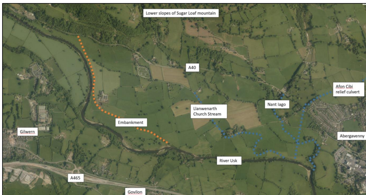
Figure 2: Llanwenarth aerial view with Main Rivers and embankment indicated.
