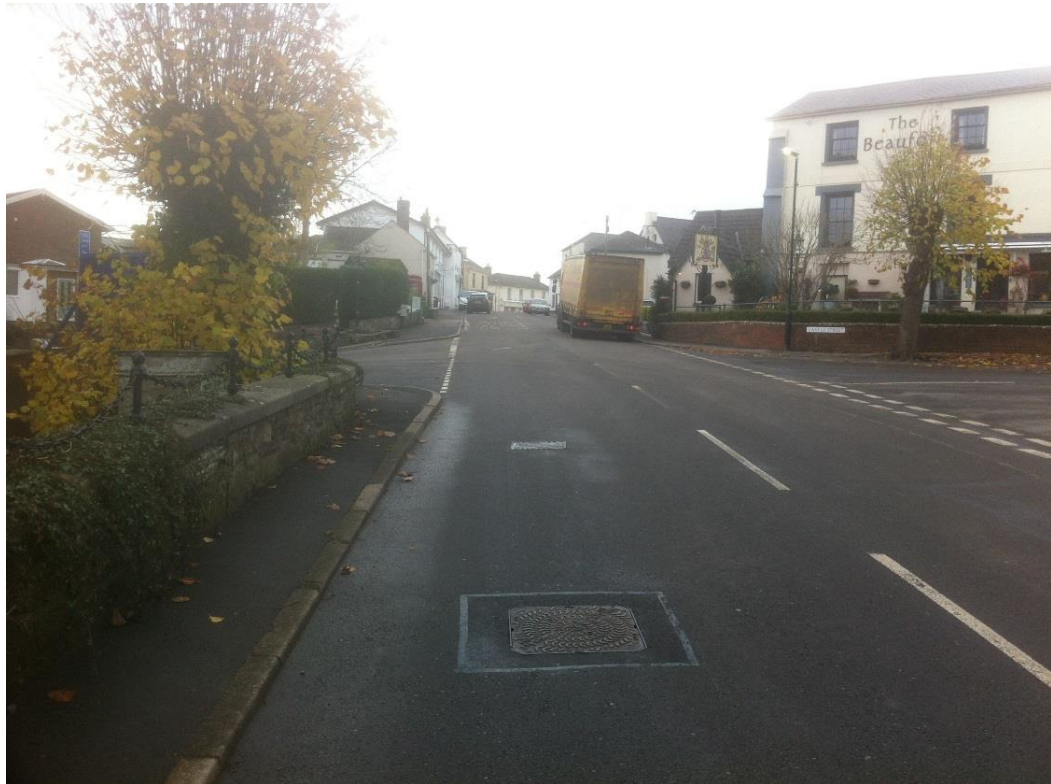
Photograph 8. Footways at Junction on Main Road / Chepstow Road
