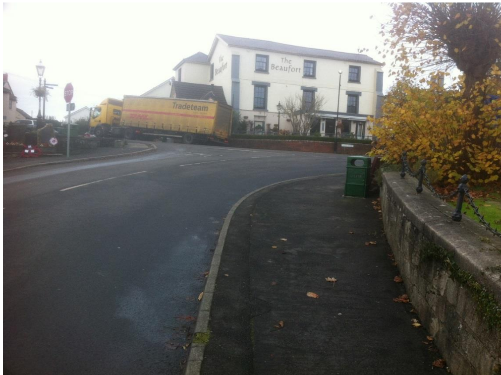
Photograph 7. Footway on Northern End of Chepstow Road leading to Main Road
