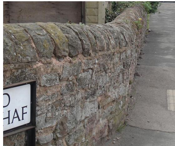
Fig.90 Boundary walls within the conservation area incorporate local stone with a distinctive half round capping
