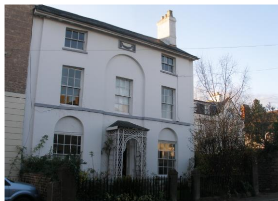
Fig.129 No. 20 Singleton House, Monk Street. A later Regency house of c 1830. The tented canopy and trelliswork of the porch offsets the formality of the overall neo-classical design.
