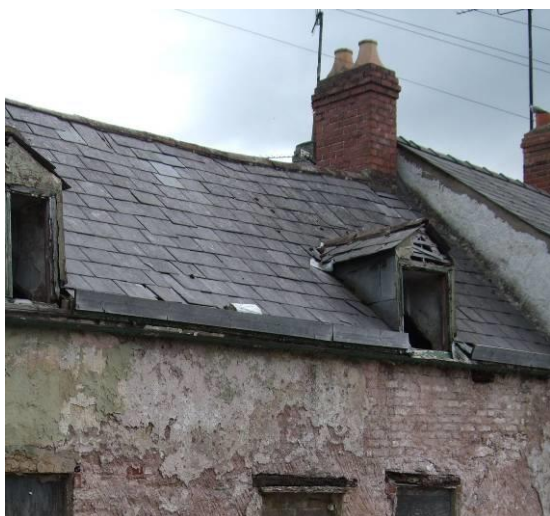
Fig.193 Natural slate is still seen to traditional buildings.
