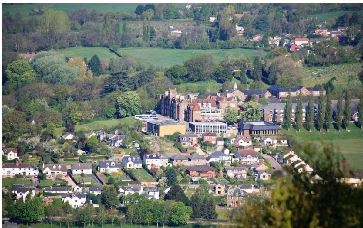
Fig.71 View from the Kymin across the town – note the dominance in scale of the school in relation to surrounding buildings (outside the conservation area)
