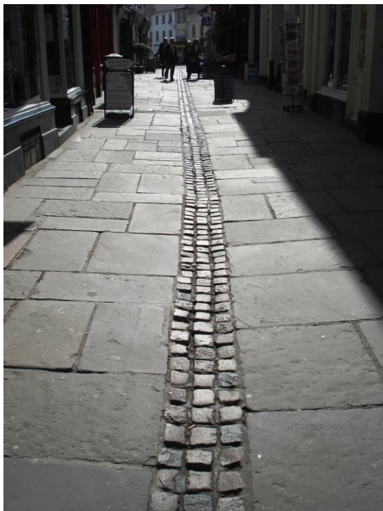
Fig.23 High quality floorscape of Pennant stone flags and central gully of small stone setts
