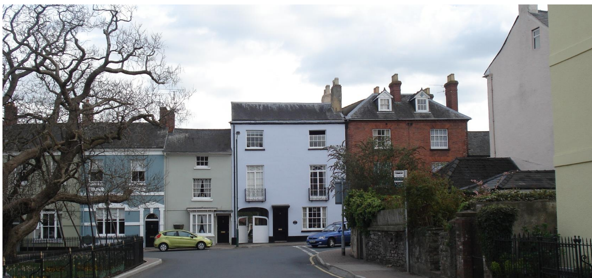
Fig.38 Architectural character around the square created by variety of well-preserved buildings of varying sizes and with painted render and brick elevations
