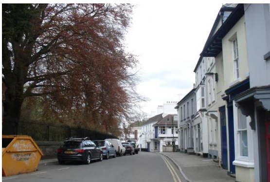
Fig.35 A view looking east along Whitecross Street showing the significant contribution that the edge of the churchyard and the trees within the churchyard make to the street.
