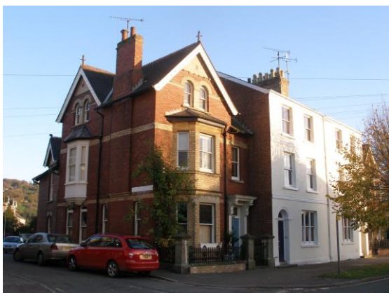
Fig.164 Westfield, on the corner of Monkswell Road, typically High Victorian domestic architecture.
