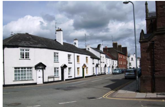
Fig.21 The terrace to the north side of Almshouse Street forms a good group of unlisted buildings to this part of the conservation area.
