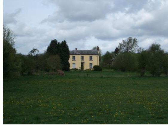
Fig.107 Vauxhall Farmhouse a prominent Grade II listed building clearly seen in extended views from the town and from across the floodplains.
