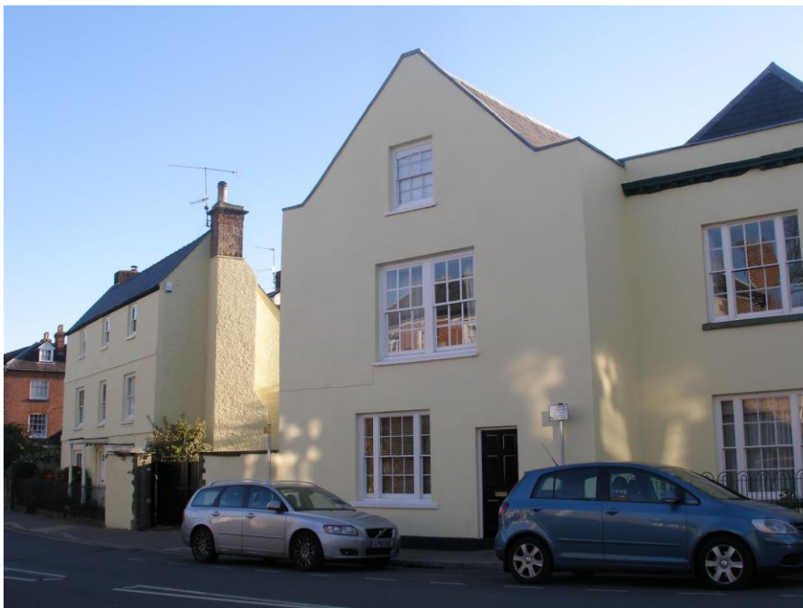
Fig.115 Nos 1 & 2 Whitecross St. The late medieval gable element of this group.
