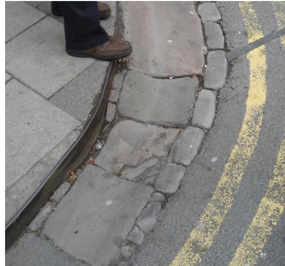
Fig.31 Pennant stone has been used locally for paving details local features significantly add to the character and appearance of the Monmouth Conservation Area
