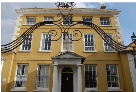
Fig.125 Cornwall House, set back from Monnow Street, behind an elegant overthrow gateway. The Doric portico is a particularly refined Georgian feature.
