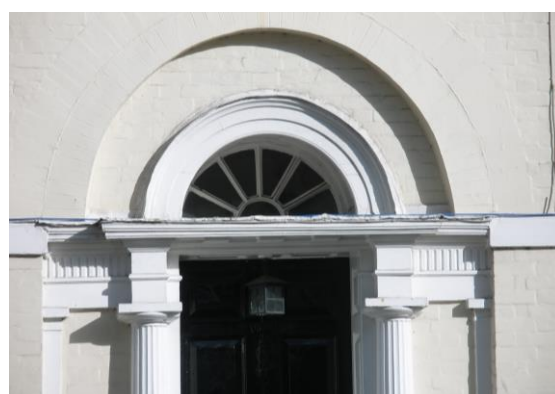
Fig.128 The refined Doric doorcase and semi-circular fanlight and recess of Chippenham House.
