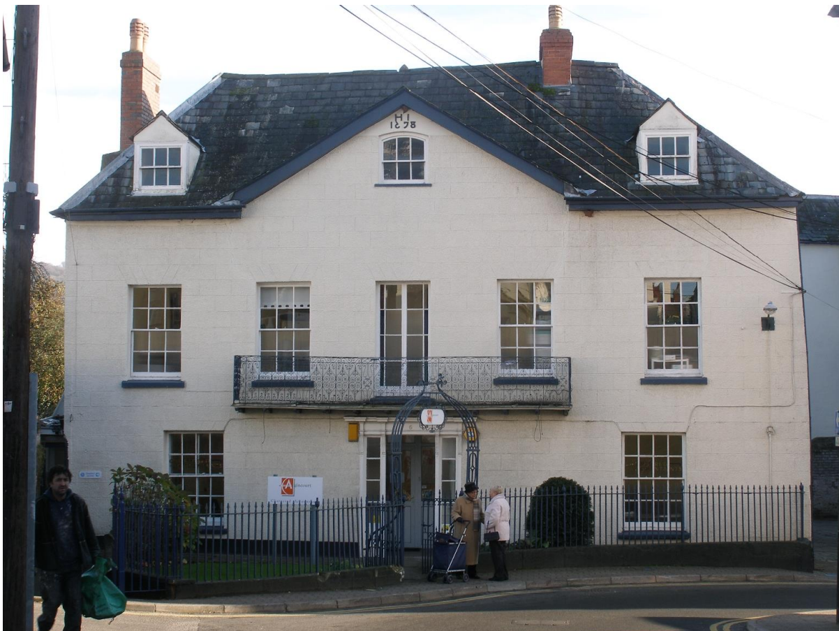
Fig.120 No 6 Agincourt Street. It is dated 1678, as can be seen in the pediment. Classical symmetry is apparent in the design, although most of the windows are later.
