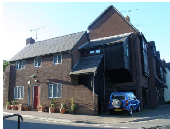
Fig.177 The Burgage, c1980s, an interesting handling of a tight corner site off Dixton Road, to create a higher density housing scheme
