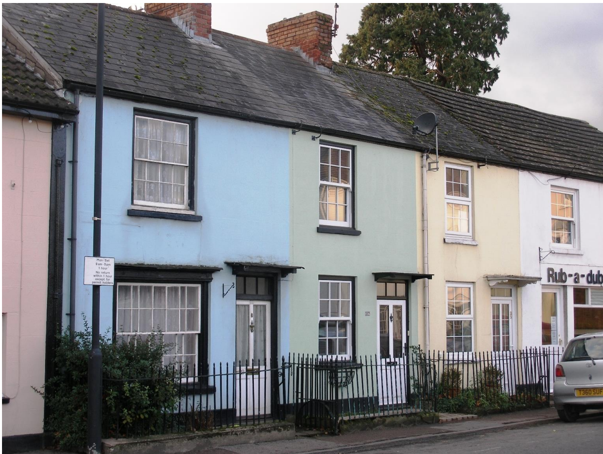
Fig.187 Cottages on Drybridge Street. These retain their sash windows in a variety of sizes.
