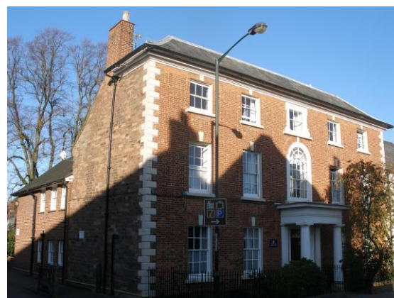
Fig.122 St James' House. Georgian refronting of a 16 th century house, as can be seen from the side.
