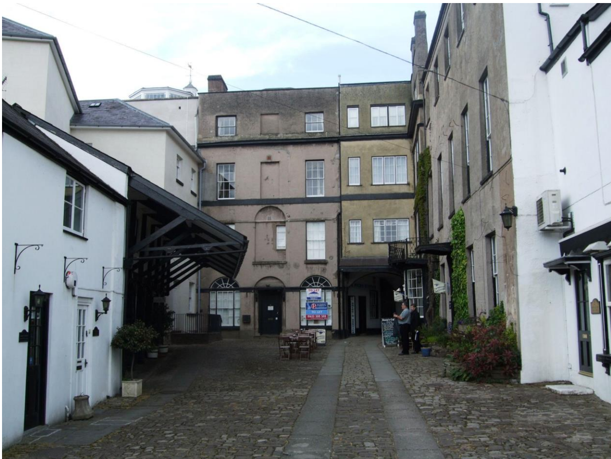
Fig.32 The courtyard to the Beaufort Arms retains its traditional stone sett surface and carriageways finished in flag stones
