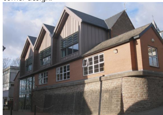
Fig.176 A recent extension at the School for Girls is a bold expression of triple gables, louvred south-facing windows and full height glazed entrance, sitting above and to one side of an existing stone wall
