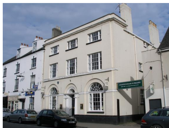
Fig.127 Chippenham House, Monnow Street, a late 18 th /early 19 th century house whose low pitched roof is typically hidden by a parapet.
