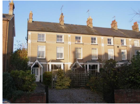
Fig.168 Nos.23-31 Monkswell Road, 1870. A simple Victorian terrace enhanced by an unusual scribing of the render and by delicate fretwork bargeboards on the canopies.
