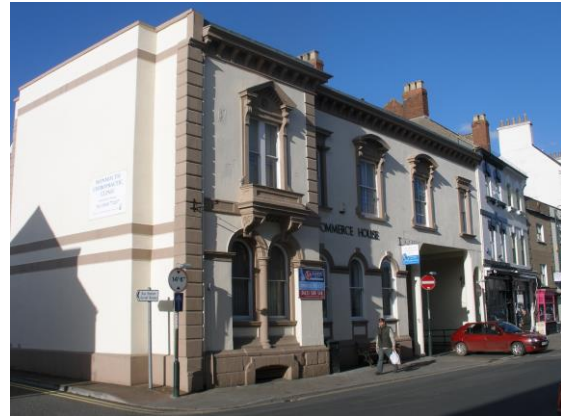
Fig.148 Commerce House at the lower end of Monnow Street retains its original Victorian Italianate characteristics on its left side, despite the drastic insertion of a roadway on its right side.
