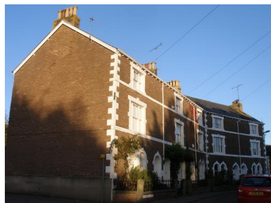
Fig.166 Nos. 1-9 Monkswell Road, built 1869, a Victorian version of the Georgian terrace, effectively following the curvature of the street.
