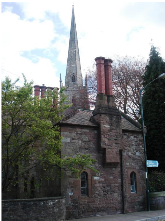
Fig.33 The spire of the church of St Mary dominates the skyline within its immediate semi-open setting to Priory Street
