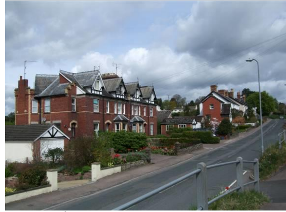
Fig.204 19 th century terrace on Hereford Road
