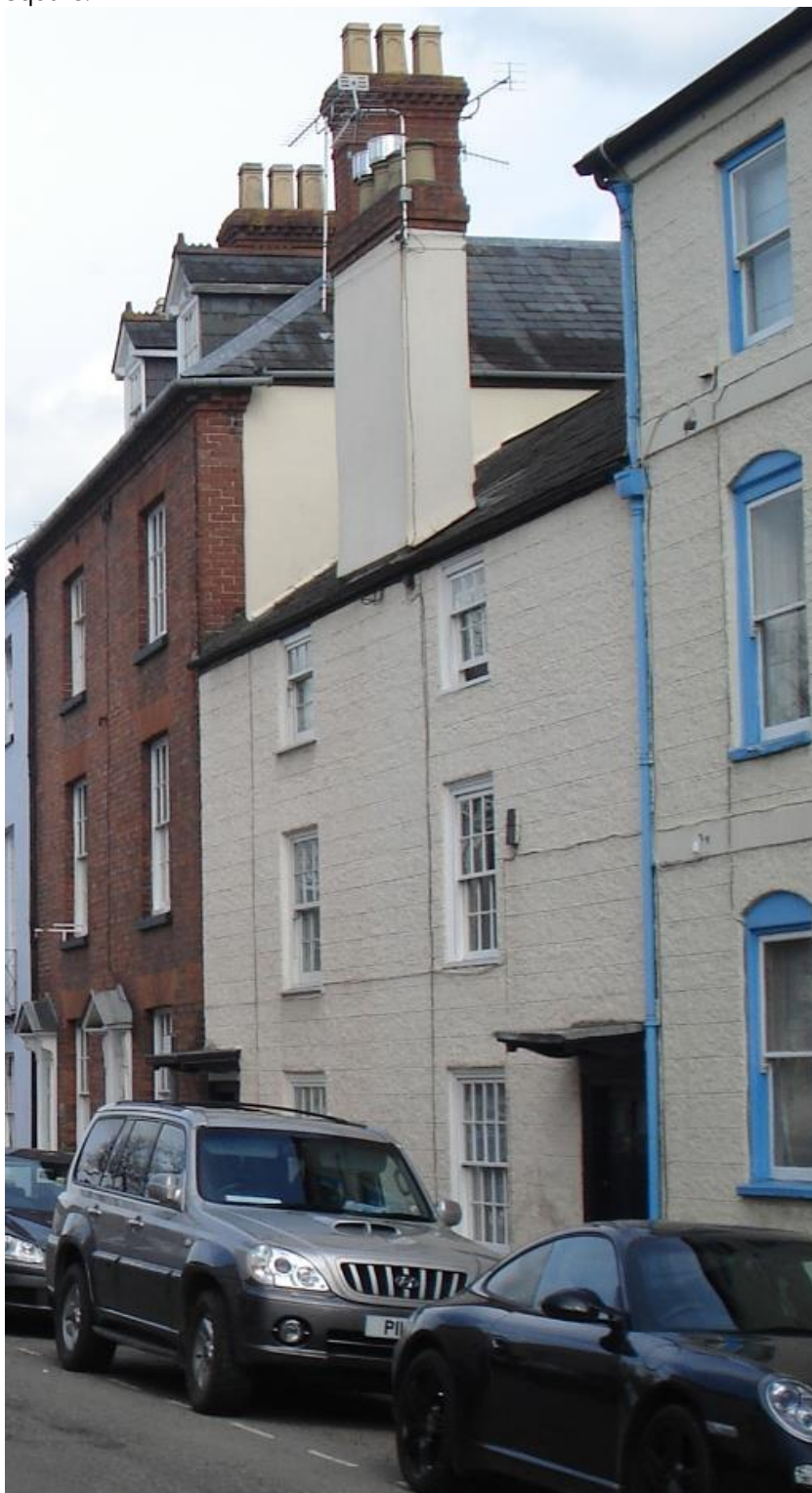
Fig.48 The unusual planting of a chimney stack to the eaves line of a principal façade seen here to a house in St James' Street
