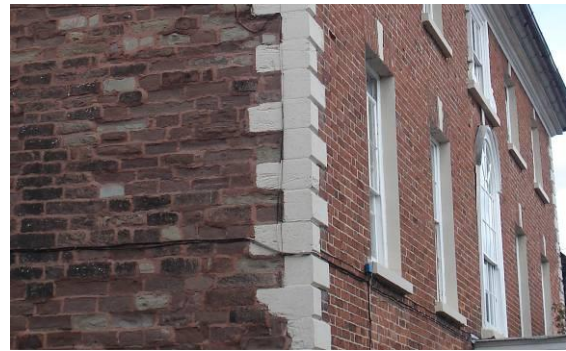
Fig.192 St James' House, a 16 th century stone building re-fronted in brick in the 18 th century.
