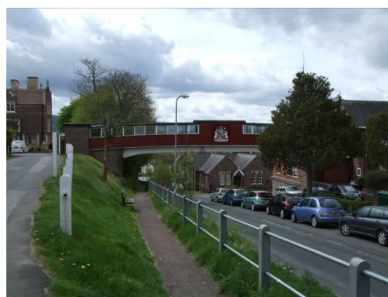
Fig.72 The pedestrian bridge linking school sites either side of the Hereford Road and acting as both local landmark and informal gateway to the town from the north
