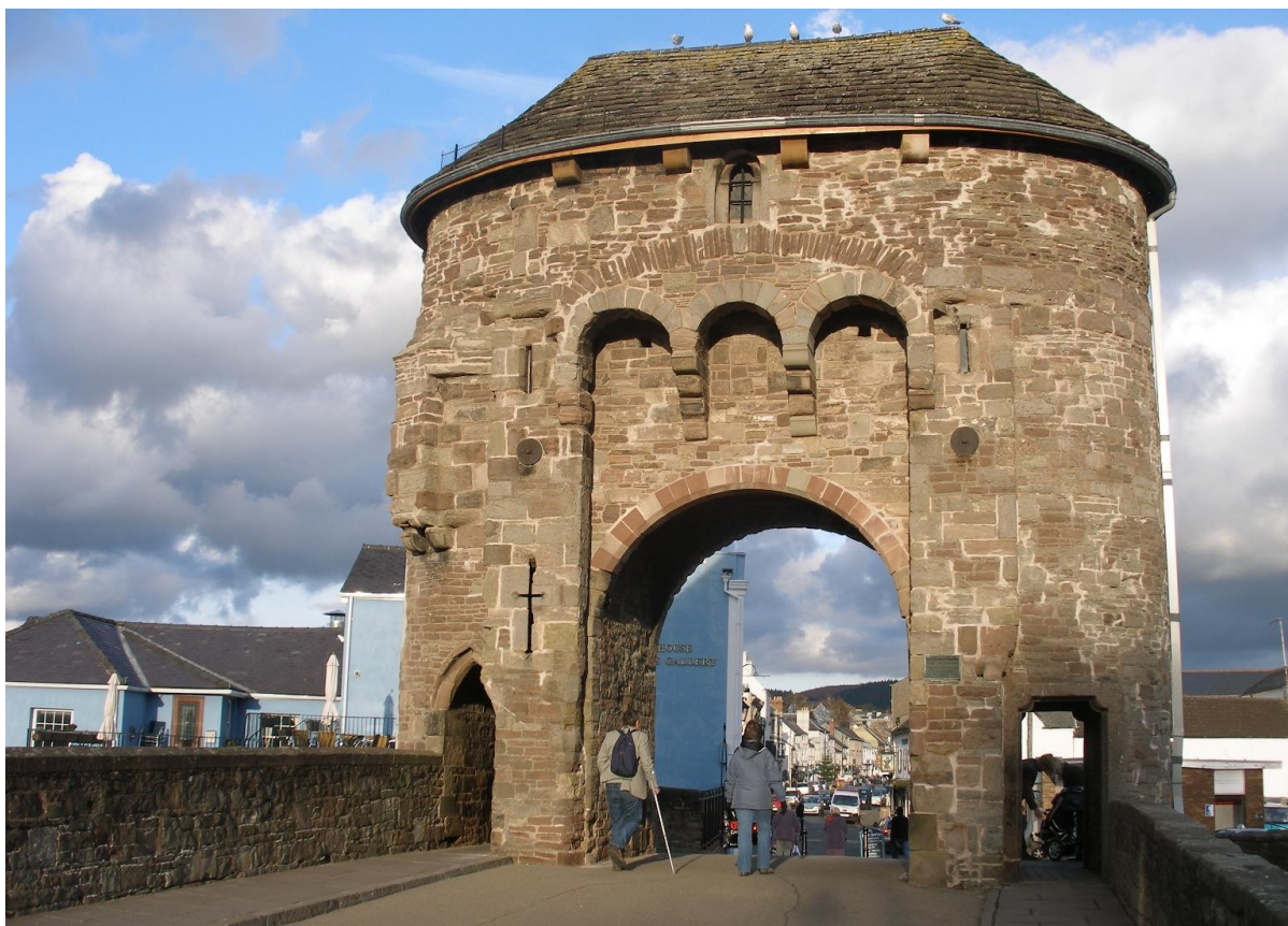
Fig.112 The Monnow Bridge Gateway is unique in Great Britain. It was built in the late 13 th century and was restored in the 19 th century.
