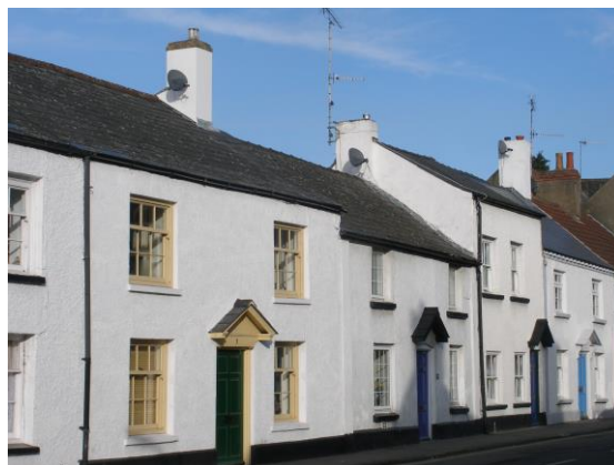
Fig.178 Well maintained vernacular cottages in Almshouse Street
