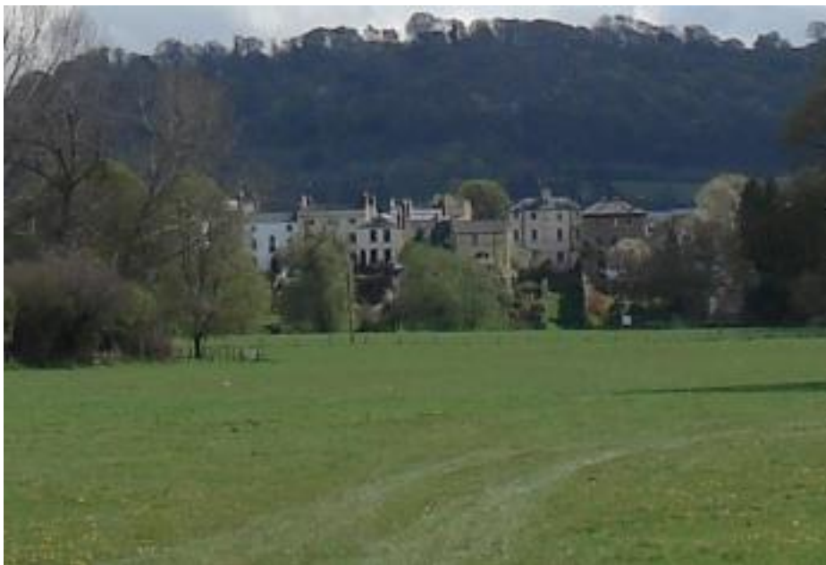
Fig.108 The rear elevations of houses to the west side of North Parade are prominent in views from the River Monnow flood plain.
