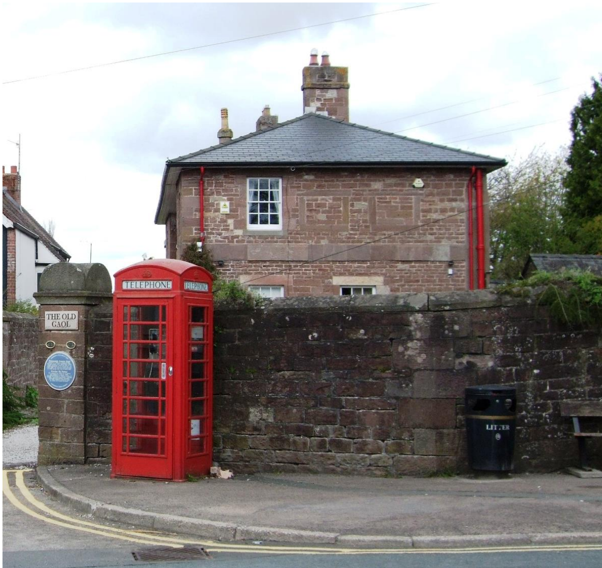
Fig.102 The gatehouse to the former County Gaol. The use of Old Red Sandstone blocks clearly defines the original window configuration on this building. The Gaol Gatehouse and its high stone wall form a good group
