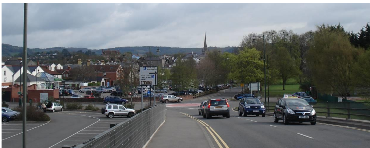
Fig.197 Views into Monmouth from the 2004 road bridge over the Monnow. The roofline of Great Castle House and the spire of St Mary's Church are landmarks set against the distant hills.
