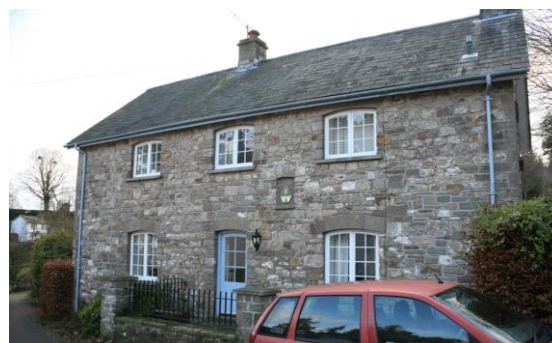
Fig.57 Rhyd-y-Meirch. A larger cottage situated parallel and behind the Post Office terrace. The skilful use of stone voussoirs forming elliptical arches over the window heads is apparent.
