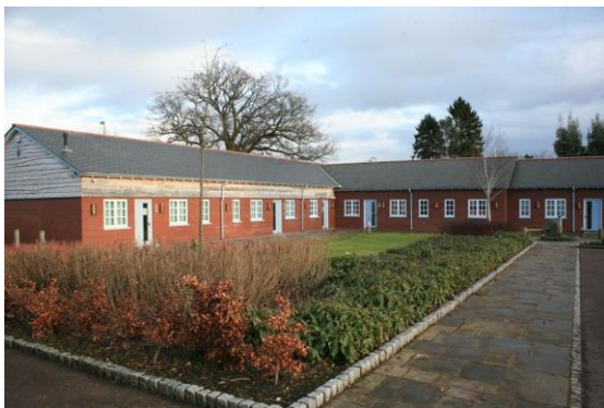
Fig.35 The new Waddington House range making up one side of the Llanover Business Centre
