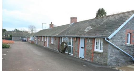
Fig.38 The rock-faced stone Treowen range to the south-west side of the courtyard group
