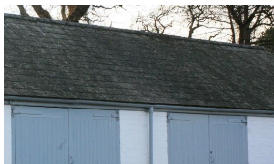
Fig.72 Cement-fibre slates are increasingly seen as natural slate is replaced or on new build
