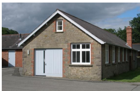
Fig.62 Former Estate Yard building. The logical and sympathetic choice of materials, good proportions and good use of colour, make this group both attractive and functional.
