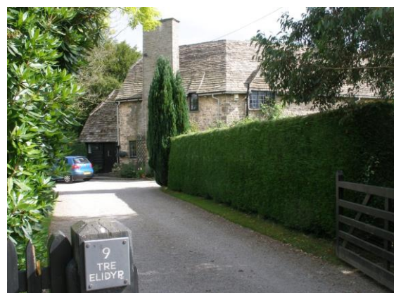
Fig.66 No. 9 Tre Elidyr. One of a pair of cottages at the northern edge of the green. The 'cranked' plan helps to enclose the green. The chimneys are significant architectural statements on such modest buildings and form an important part of the composition of the houses.
