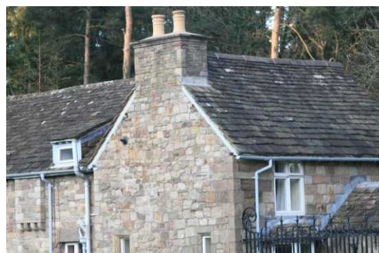
Fig.71 Richly coloured stone slates are seen to buildings throughout the Conservation Area
