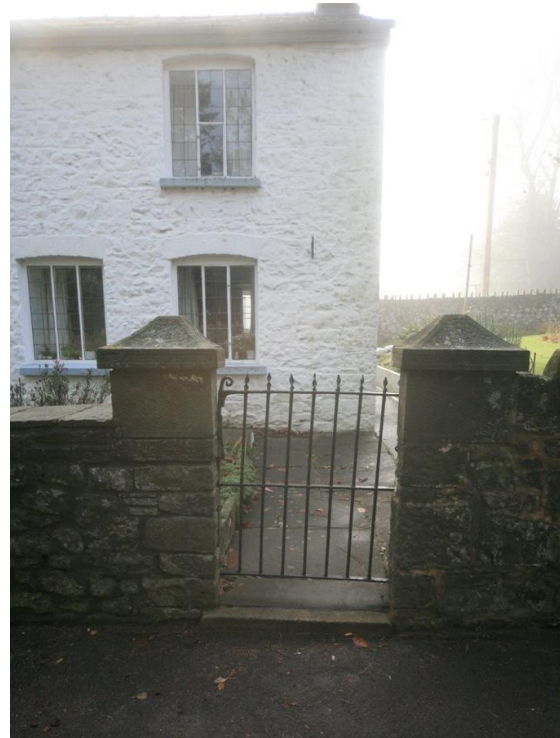
Fig.54 Stone gate piers and iron gate to Laburnham Cottages
