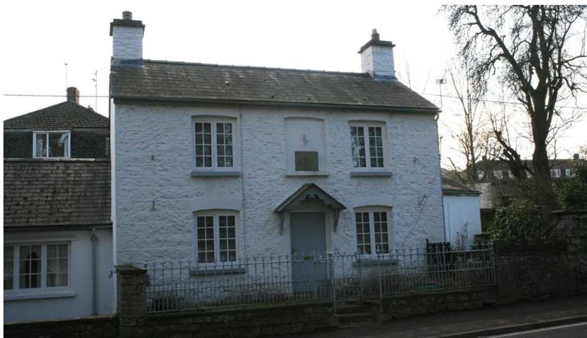
Fig.58 Y Llyth-yr-dr Cottage. This nearly symmetrical cottage demonstrates the generally higher standard of design characteristic of estate cottages. The scrolled bargeboard to the porch is an attractive feature, as are the iron railings.
