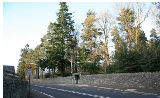
Fig.45 The park boundary wall dominates and strongly defines this part of the Conservation Area
