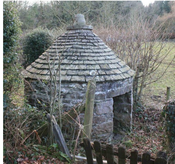
Fig.60 Circular pigsty, restored, in the garden of Well Cottage, Rhyd-y-Meirch. The use of stone in its conical roof is particularly skilful.
