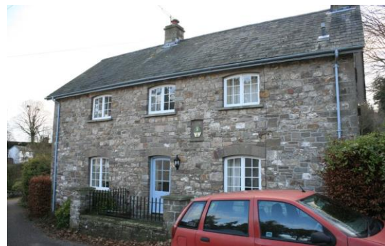
Fig.15 An example of exposed rubblestone in the character area at Y-Gwesty Stables
