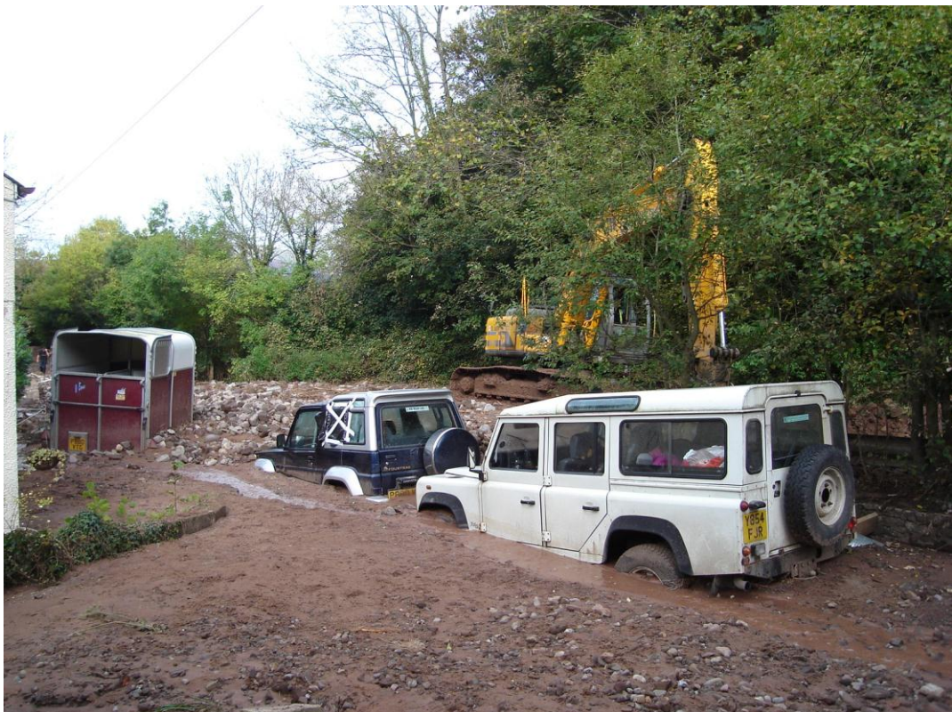
Fig 3.1 Canal Collapse at Gilwern, 2007.
