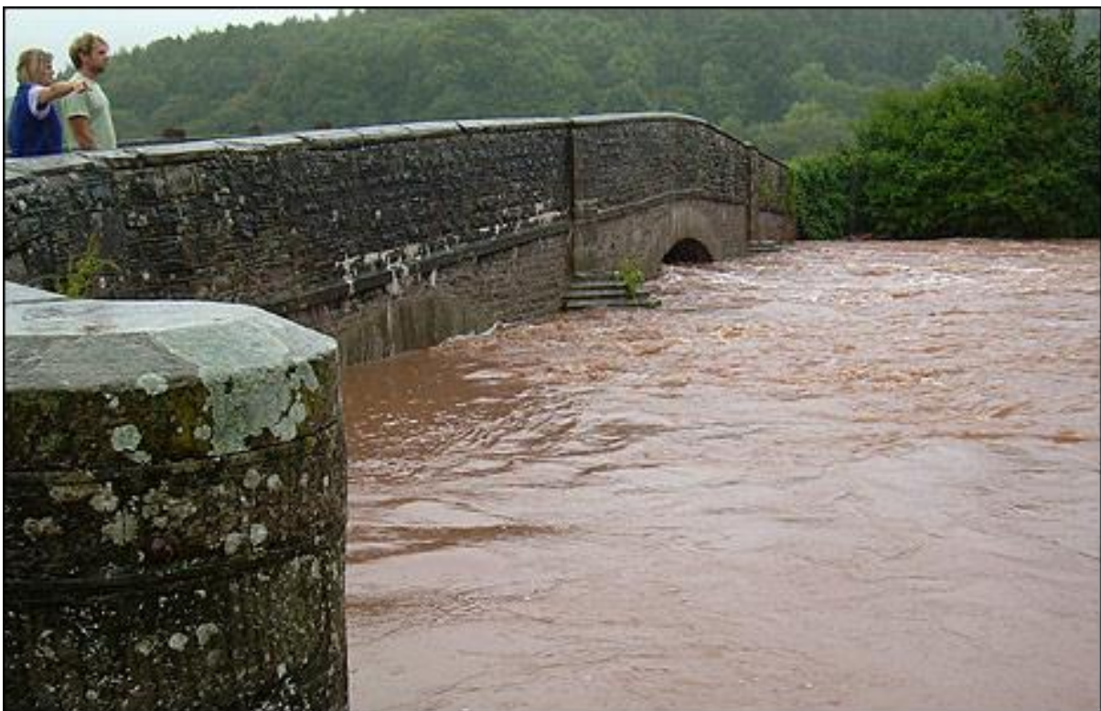
Fig 4.1 Example of Main River Flooding in Monmouthshire
