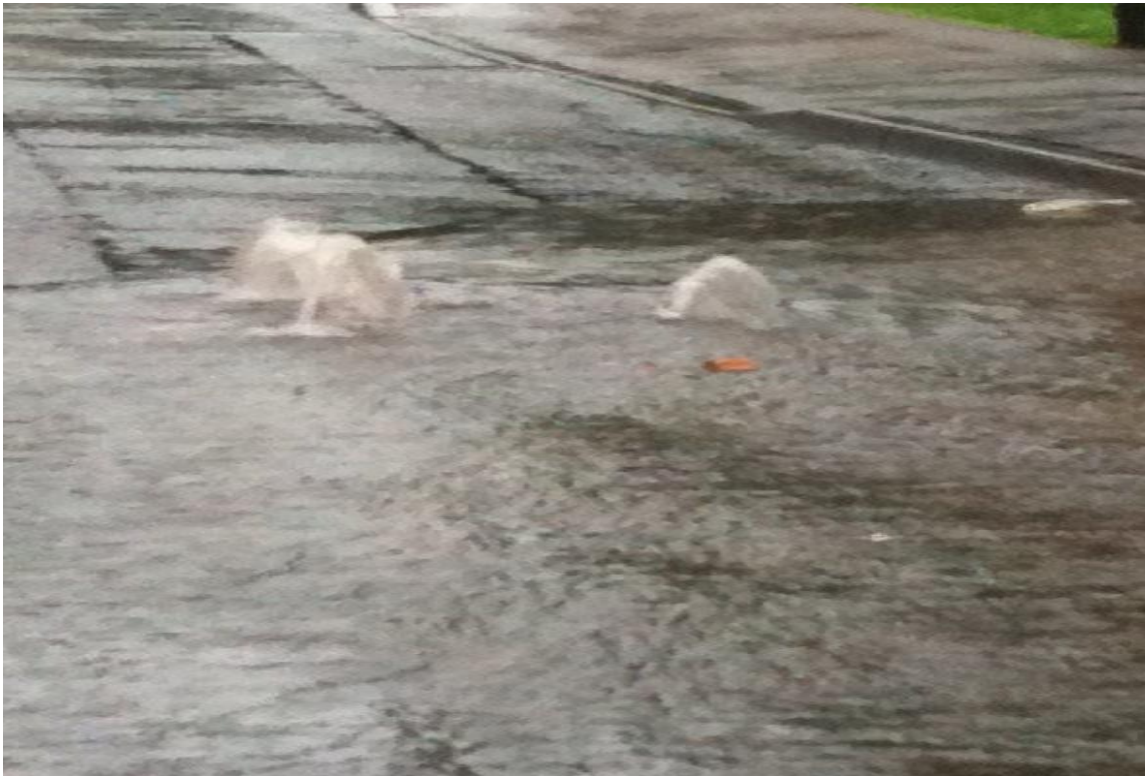
Fig 2.1 - Highway Flooding at Llanfoist after Heavy Rainfall
