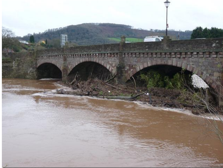
Debris Build up on Wye Bridge, Monmouth
