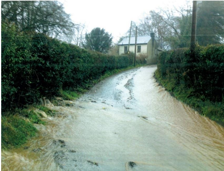
Surface Water Runoff & Carriageway Flooding, Llanvair Kilgeddin
