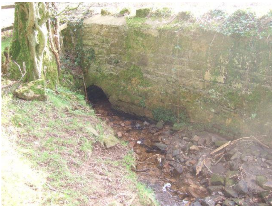
Masonry arch conveying unnamed watercourse beneath Devauden Road
