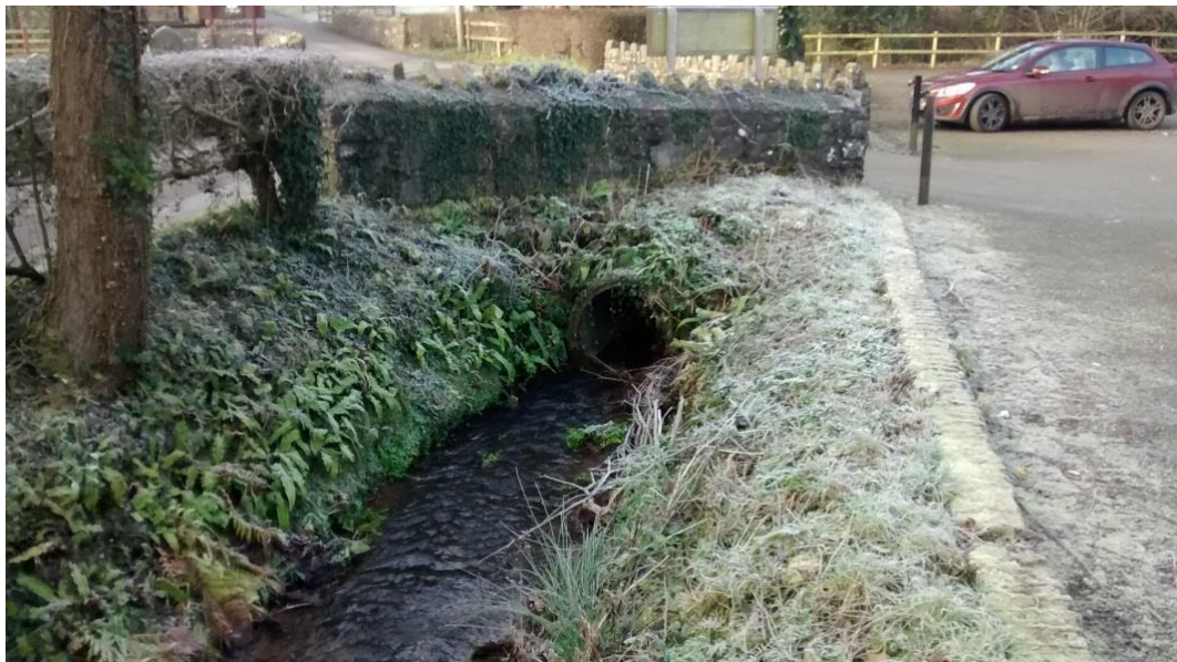
Ordinary Watercourse & Culvert at St Teilio's Church
