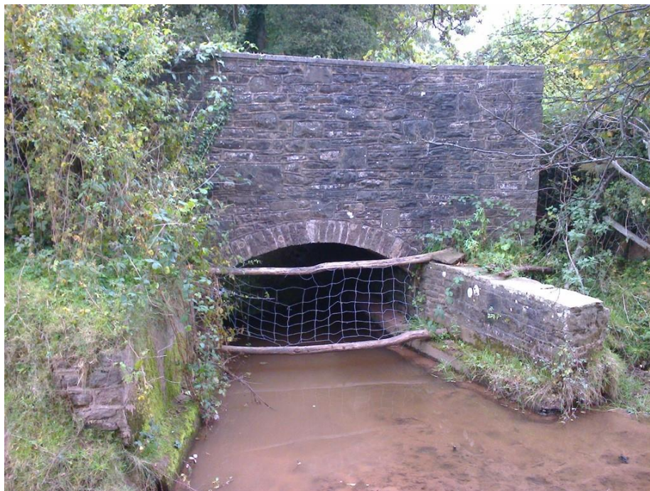
Masonry arch over the Pill Brook
