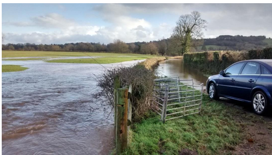
Surface Water & Carriageway Flooding near Pant-y-goitre
