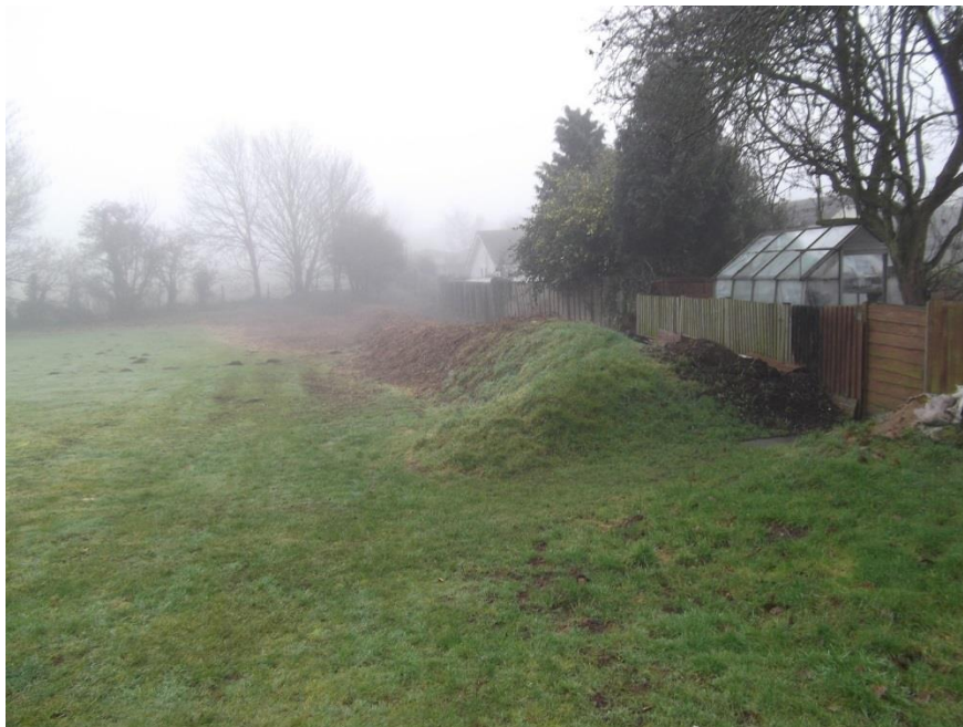
Flood bund north of Main Road
