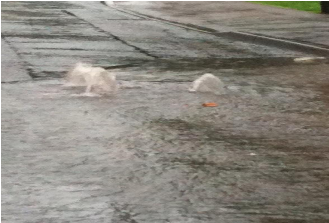
Fig 2.1 - Highway Flooding at Llanfoist after Heavy Rainfall
