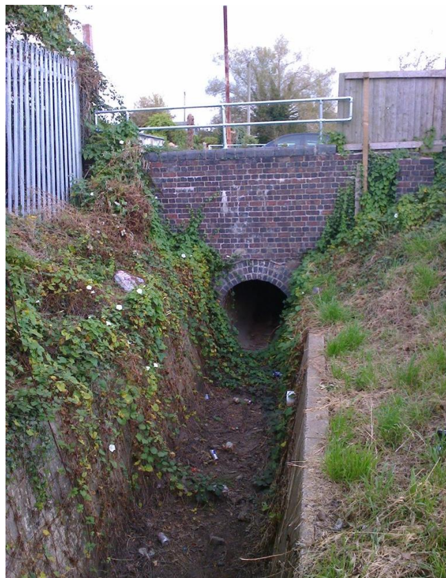
Culvert under station access road
