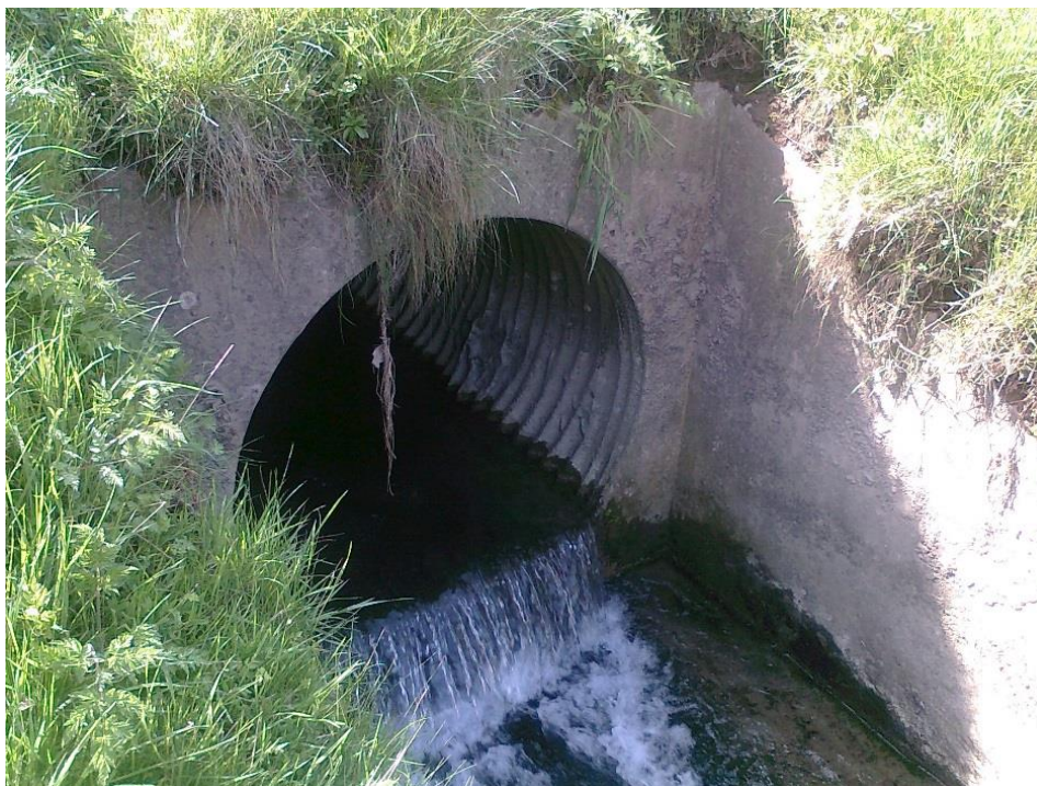
Ordinary Watercourse Outfall to River Usk at Llanbadoc Church
