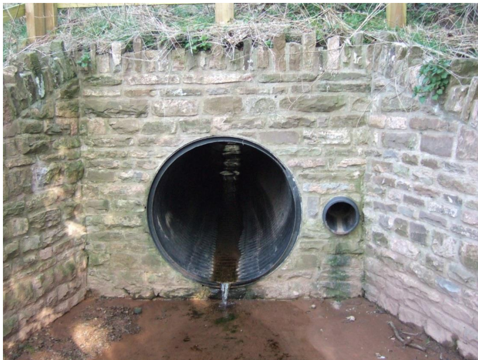
Culvert on unnamed watercourse
