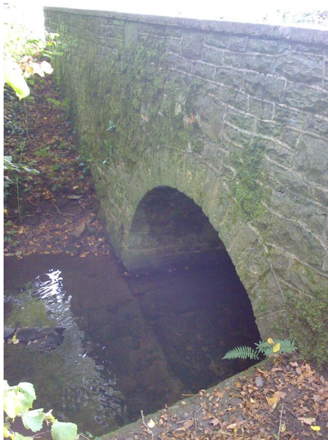
Masonry arch bridge over the Mounton Brook
