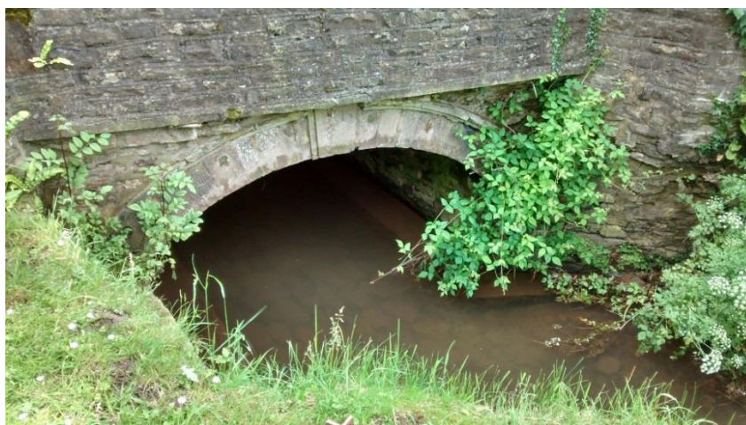
Masonry Arch Bridge over White Castle Brook
