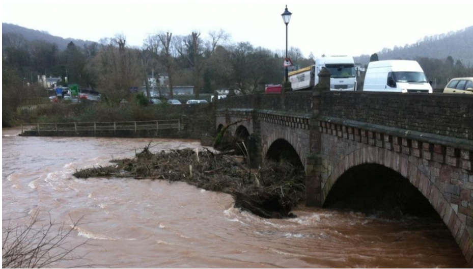
Debris Accumulations at Wye Bridge in 2013 /14
