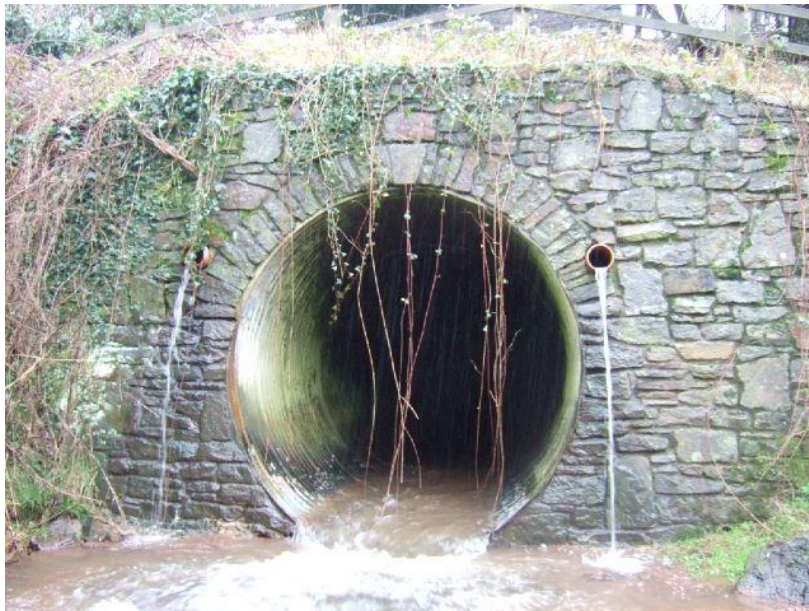
Culvert beneath the B4235
