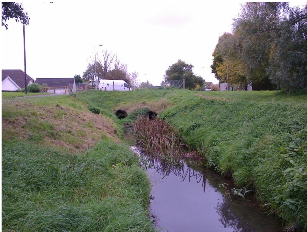
Twin culvert on the Mill Reen
