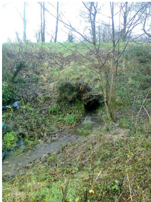
Croes-y-Pant – culvert outlet beneath Monmouth & Brecon Canal. Canal
