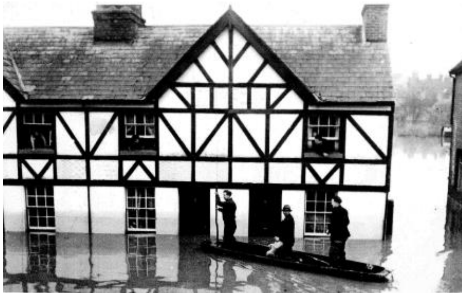
Flooding at Drybridge Street, 1947
