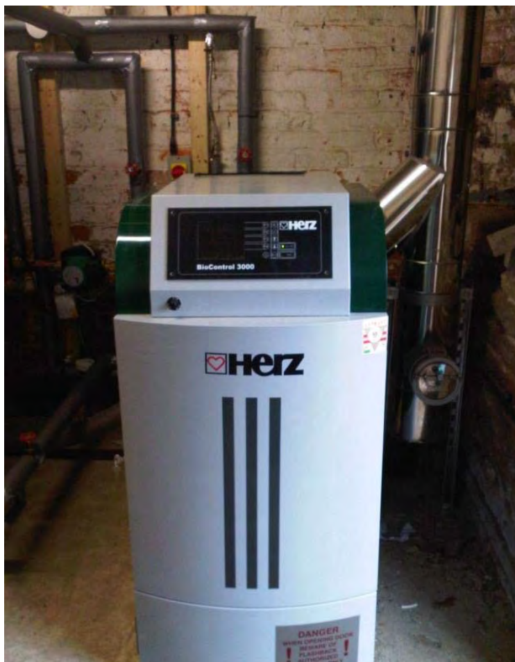
Domestic scale biomass boiler
