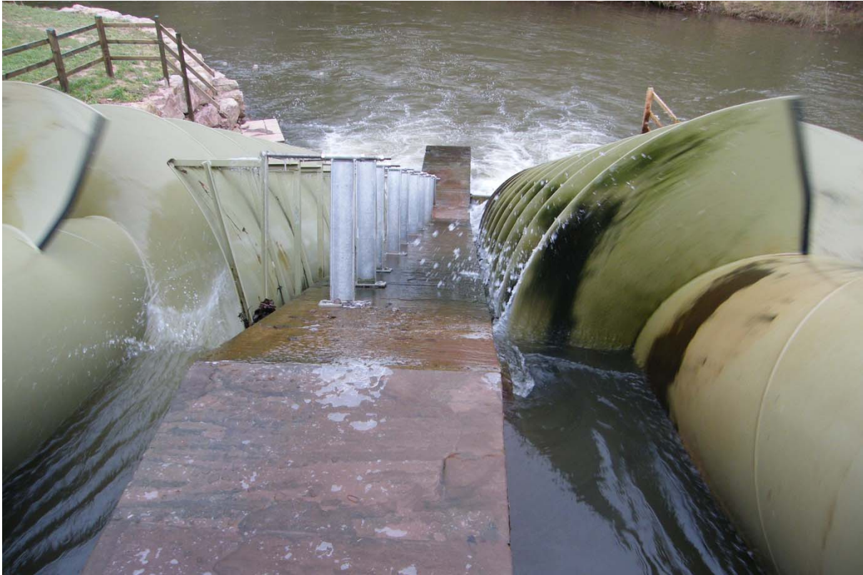
Osbaston Hydro project, Monmouthshire – Archimedes screw system Image source: Monmouthshire County Council
